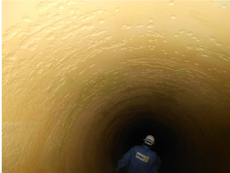
Figure (d): After primer is coated (Original in colour)
