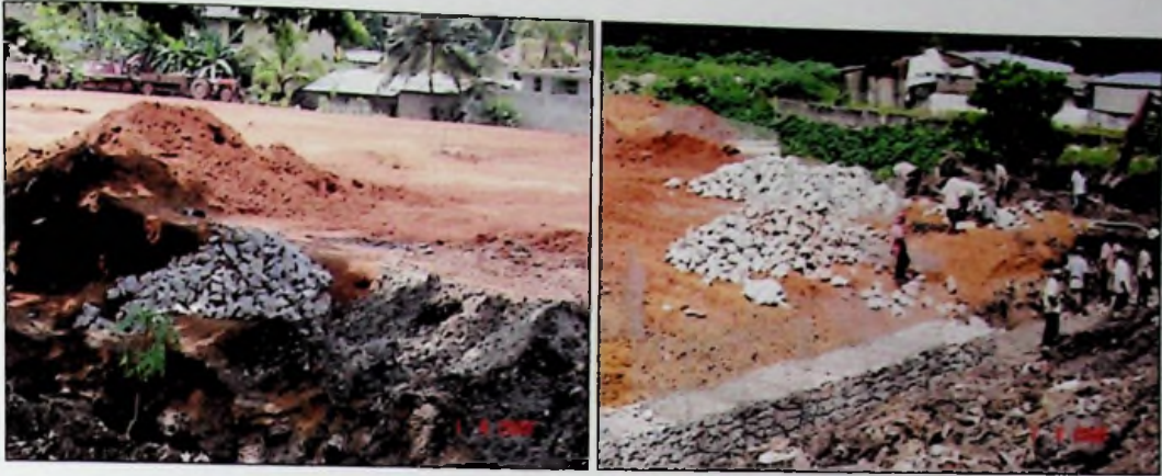
Figure 4.17 Rehabilitation of the dump site in progress, construction of retaining walls
