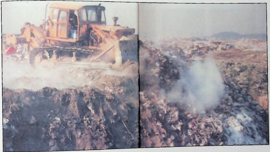
Figure 4.2: Nanjido landfill - Cover the waste with soil
