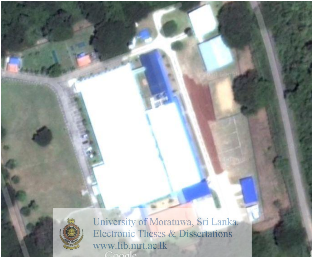
Figure:5-1: Google Image of Facility
