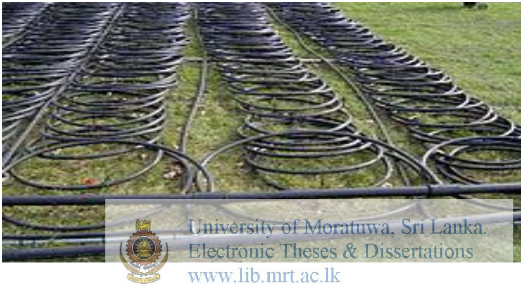
Figure 2.3 : Loop field for a 12-ton System [15]
