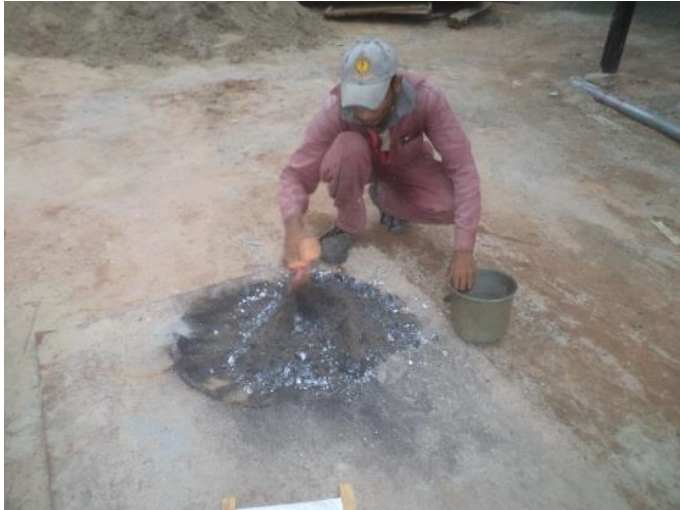
Figure 31: Mixing of charcoal, lime and sand
