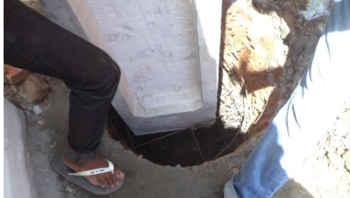
Figure 49: Planting Pole in Earth mesh
