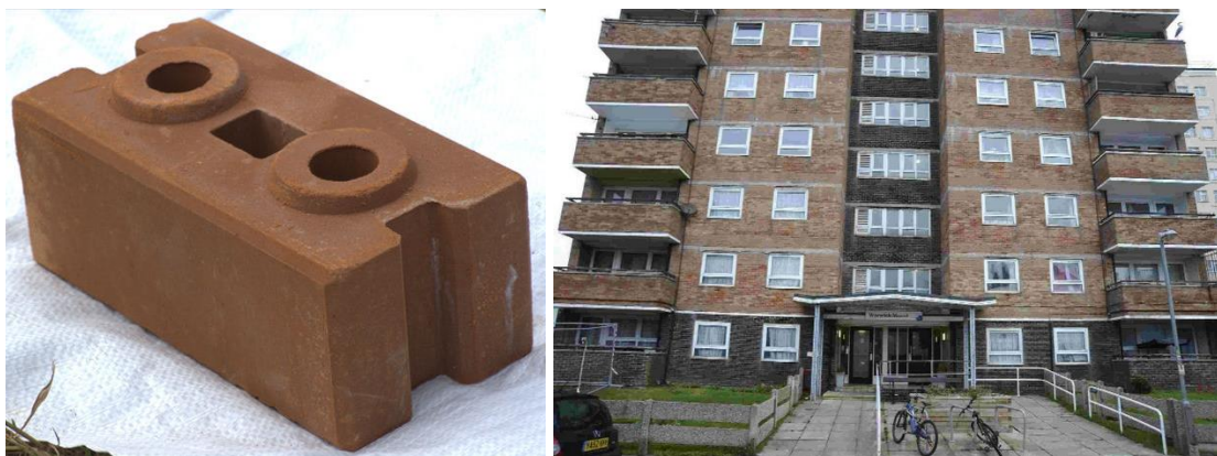
Figure 10-13: A CSEB block (left) and a building constructed with them (right)
