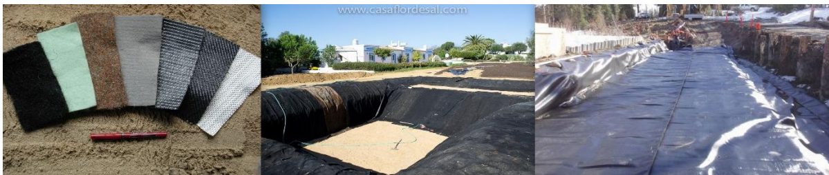
Figure 10-2: Geotextiles and their applications
