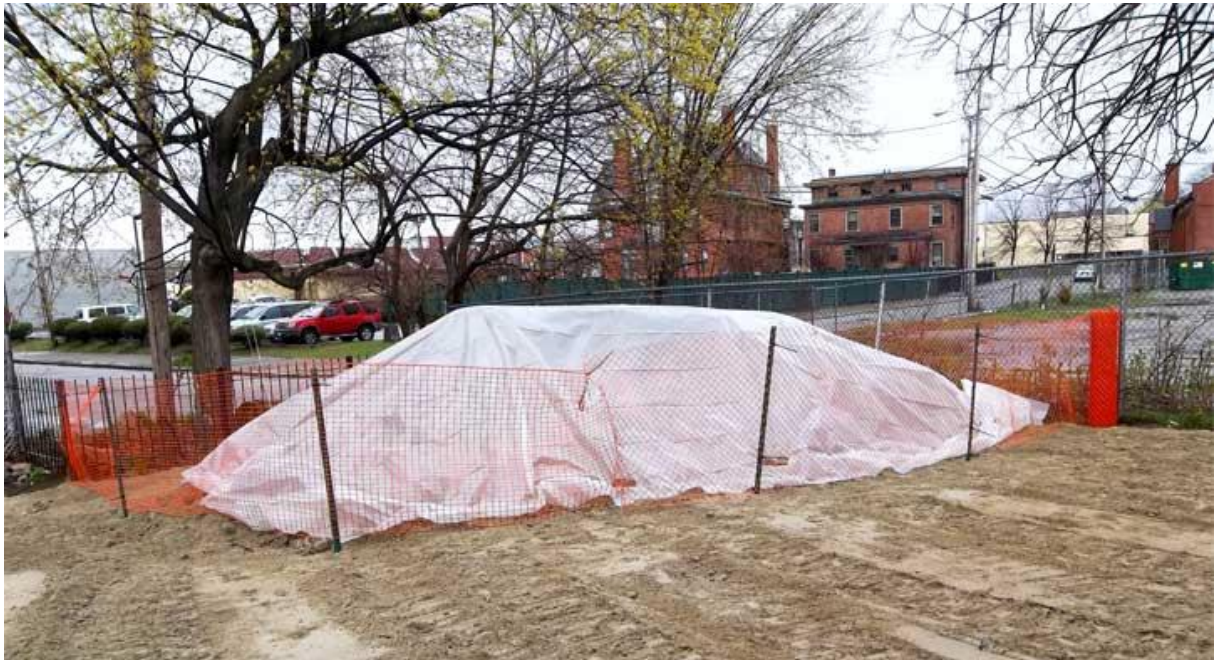
Figure 10-1: Well protected stock pile University of Moratuwa, Sri Lanka.
