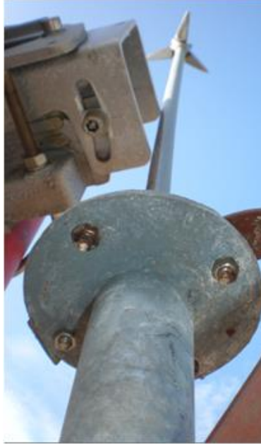
Figure 3.2: Air Terminal system
