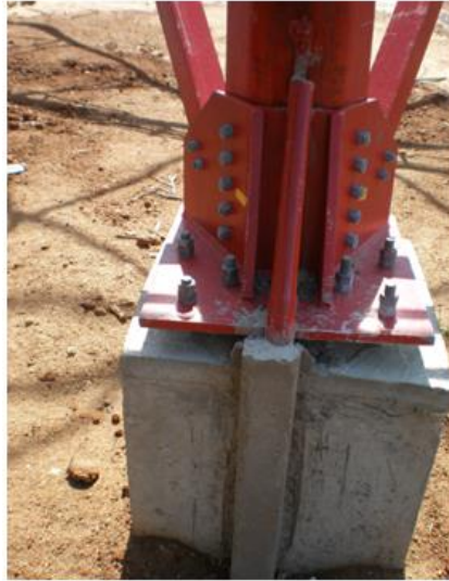
Figure 3.3: Tower structure connected to the ring earth
