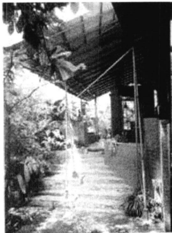
Figure 30: Thin scaffold poles supports the simple roof
