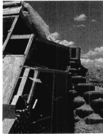
Figure 19: Michael Reynolds Earth ship made from rammed earth tires. (Source: The Everyday & Architecture)
