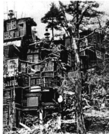
Figure 14: Squatter dwelling, Clarence Schmidt built his own house, it is kind of a log cabin, tarred, and decorated with fragments of glass refuse old windows and doorframes, old wood. (Source: 10)
