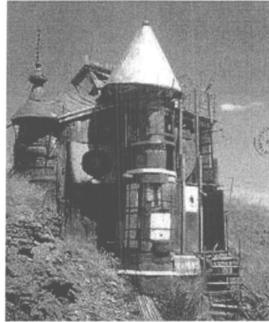
Figure 20: Victor Moore's junk castle-made out of car doors, chunks of metal from old combine machines, old bedsteads, and road signs. (Source: 10)
