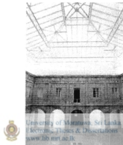
Figure 16: Reuse old building for new function. (Source: Re/architecture)
