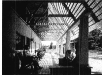
Figure 43: The skeletal roof structure enhance more lighting and openness to their social life
