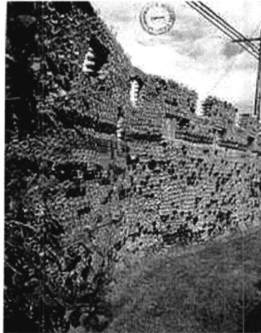
Figure 18: Garden wall made by discarded bottles. (Source: 10)
