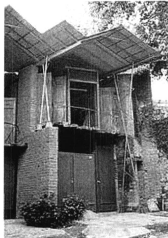
Figure 29: Front view of the house Skin of the front facade covered by the salvage door sashes
