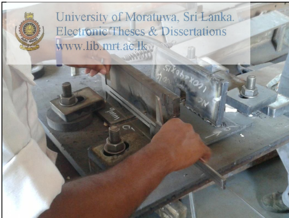
Figure 18: Taking measurements after root welding
