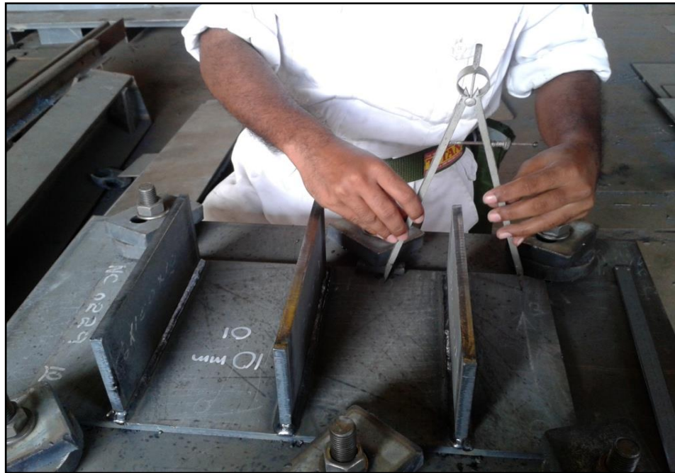
Figure 19: Taking measurements after final welding
