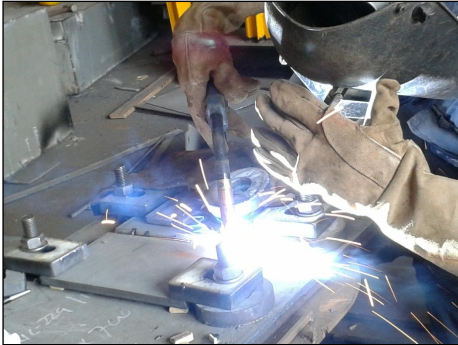
Figure 17: Carry out welding of test pieces
