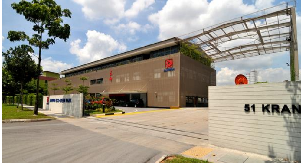
Figure 2. 6: Samwoh Eco-Green Building
