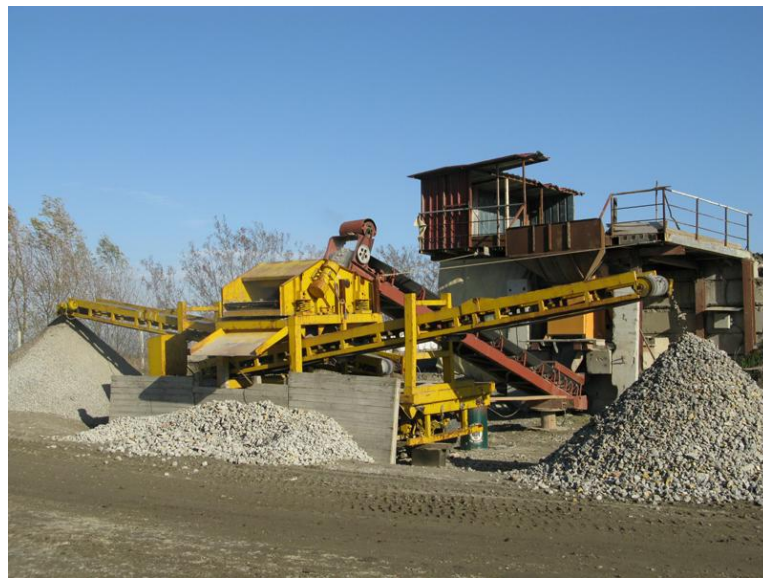
Figure 2. 12: Mobile Recycling Plant
