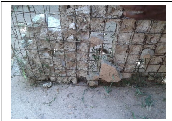
(Image 4.3.1.4 & 5: Wall Constructed using Rig form Coated GI Mesh in Malapalawatta H.S)
