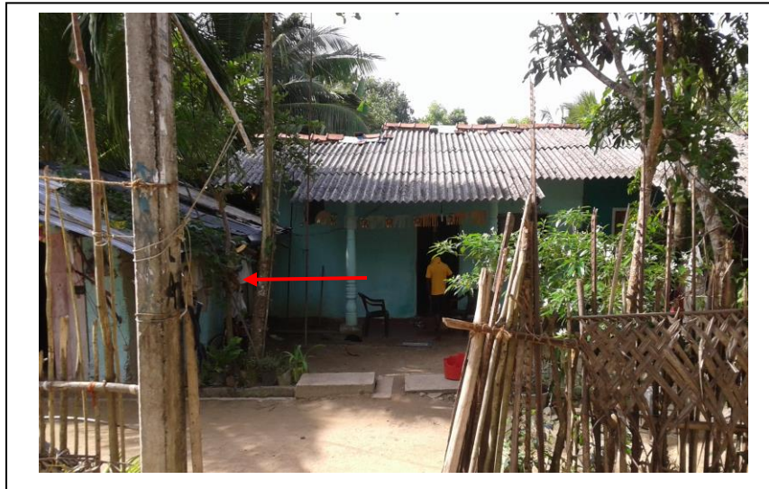
(Image 4.3.1.4: Temporary House Build in House Premise- Addunkele H.S)
