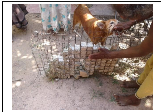
(Image 4.3.1.4 & 5: Wall Constructed using Rig form Coated GI Mesh in Malapalawatta H.S)
