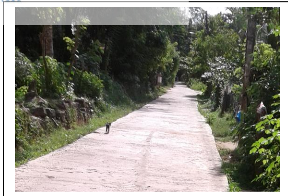
(Image 4.3.1.5 & 6 : Not Backfilled Road sides in Addunkele H.S)
