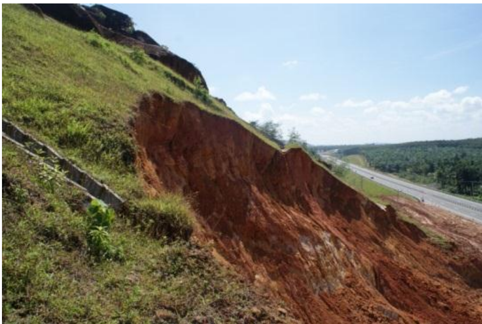
Figure 2.7 : Whitish zones encountered in a failure mass
