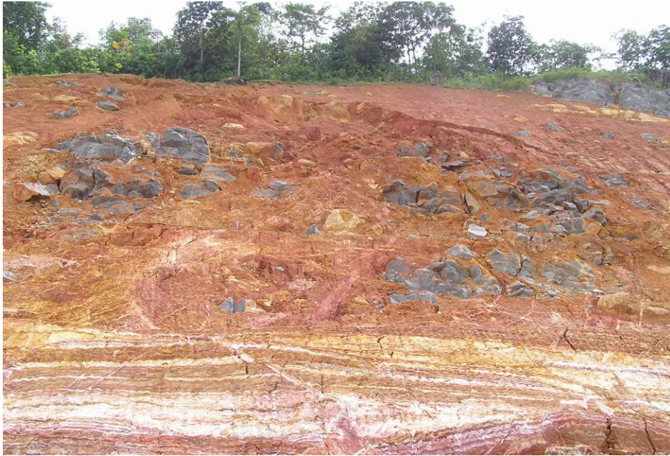
Figure 2.6: Degree of Weathering and the Nature of the weathered product varies within a short distance
