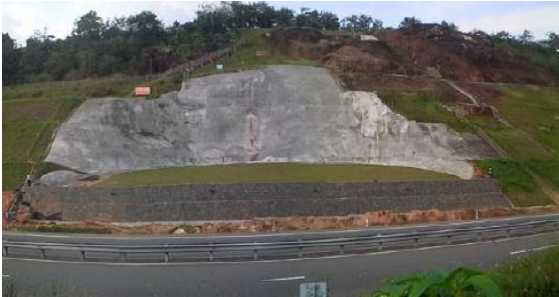
Figure 3.16: View after completing the rectification (After Dharmasena et.al 2015)
