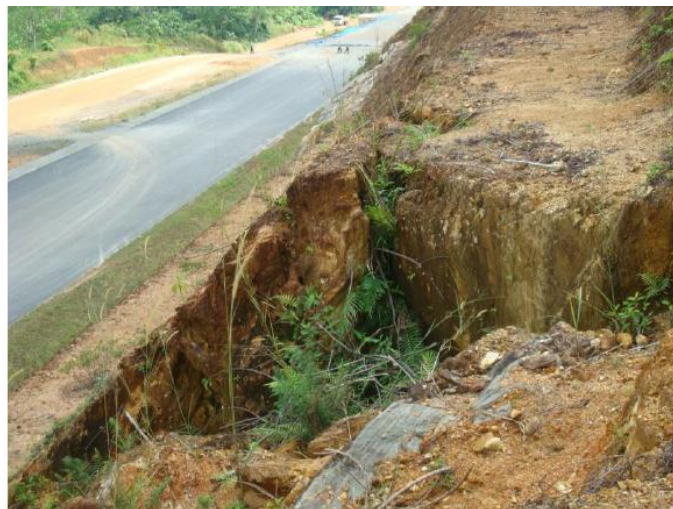
Figure 2.9: Toppling (Fall) Mode of failure could take place through relict joints
