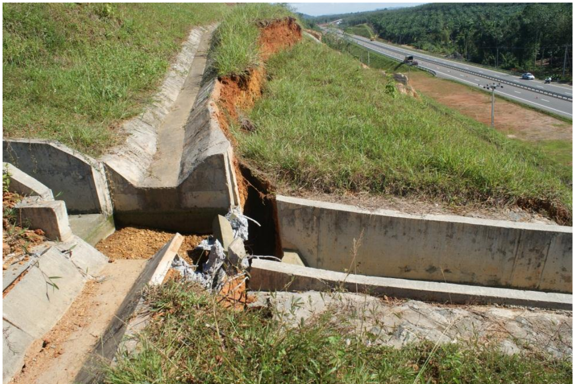
Figure 3.9– Movements of soil at the top and Movement of Cascade Drain
