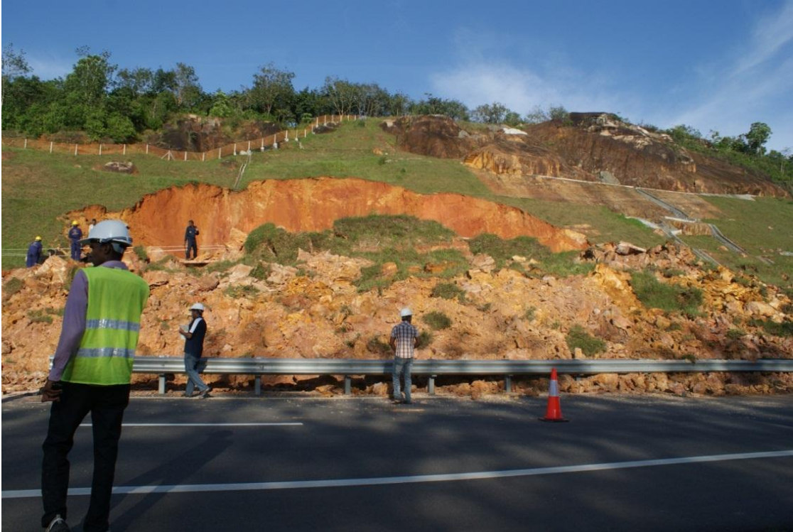
Figure 3.10– Debris of Failure Has Covered the road section towards the Galle
