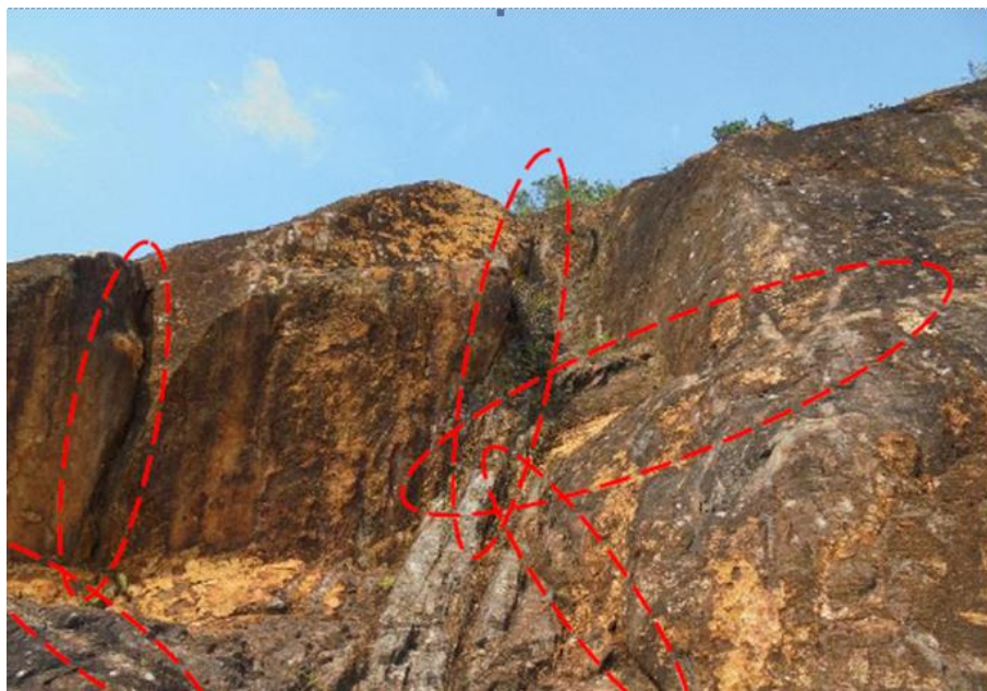
Figure 3.2 – Joint sets in the bedrock exposed at the top of the slope
