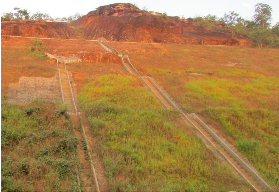
Figure 3.7: Berm drains and cascade drains
