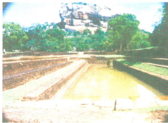
Fig 3.7 – Sigiriya, Lowest Garden. Long rectangular stepped pool to maintain display as water level drops.
