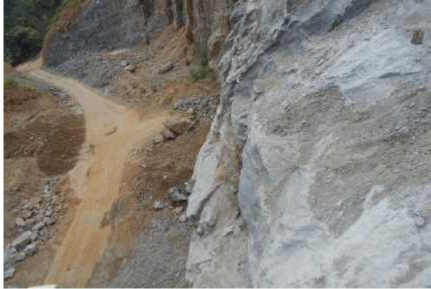
Figures 3.1 Image of cleared zone before blast
