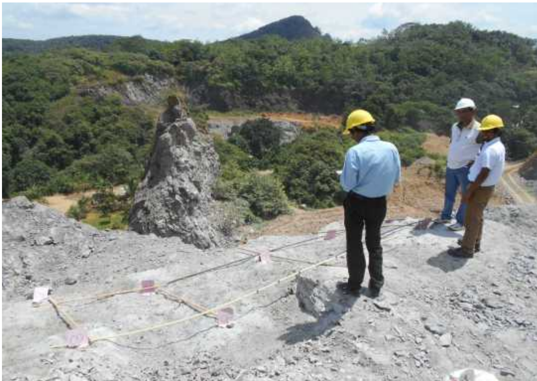
Figure 7.33: Arrangement of bore holes in phase 10
