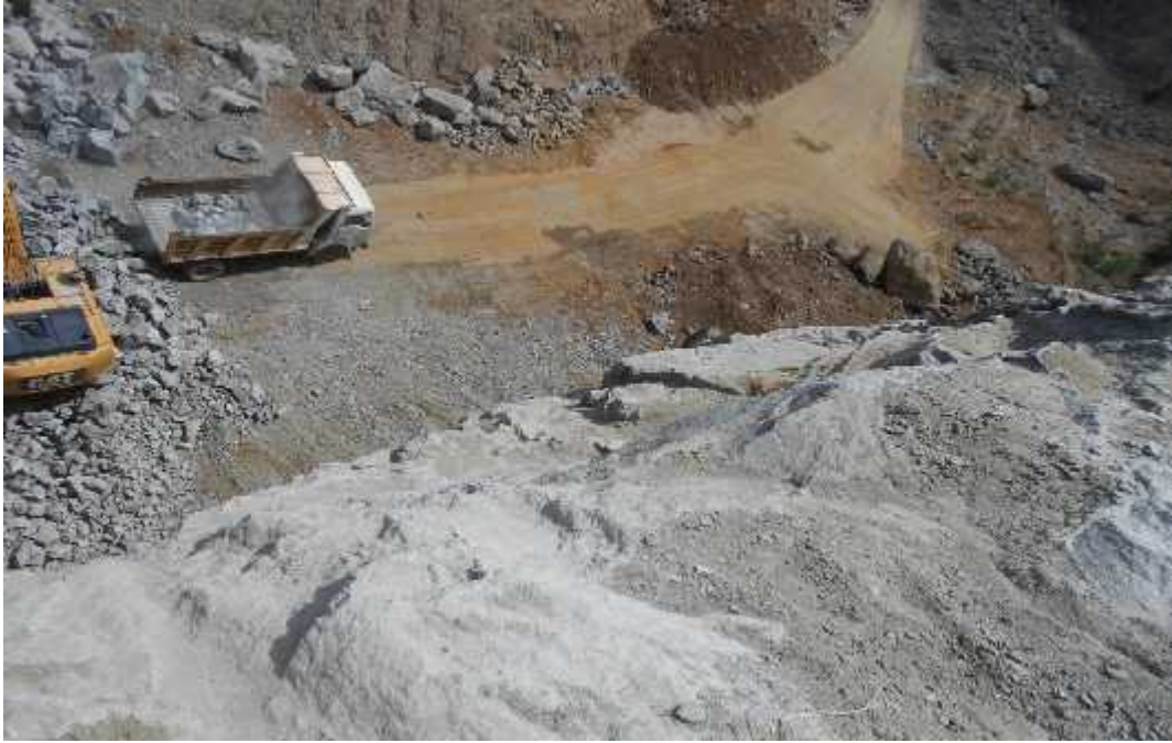
Figure 7.41: Cleared area which is expected to receive the products of blasts
