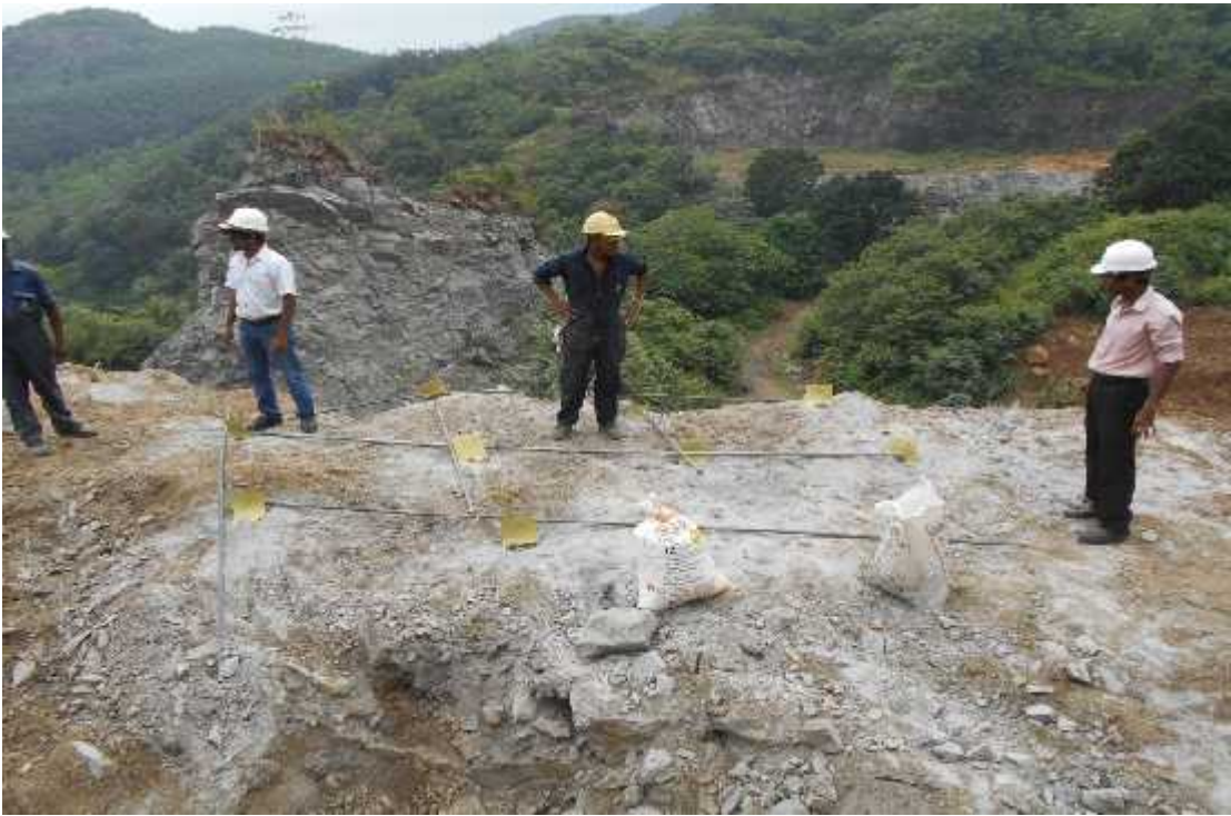
Figure 7.6 Arrangement of bore holes in phase 2
