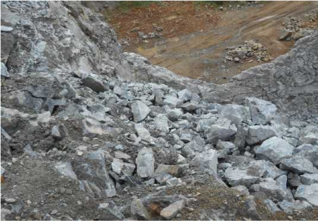
Figure 7.4: After the blast in phase 1
