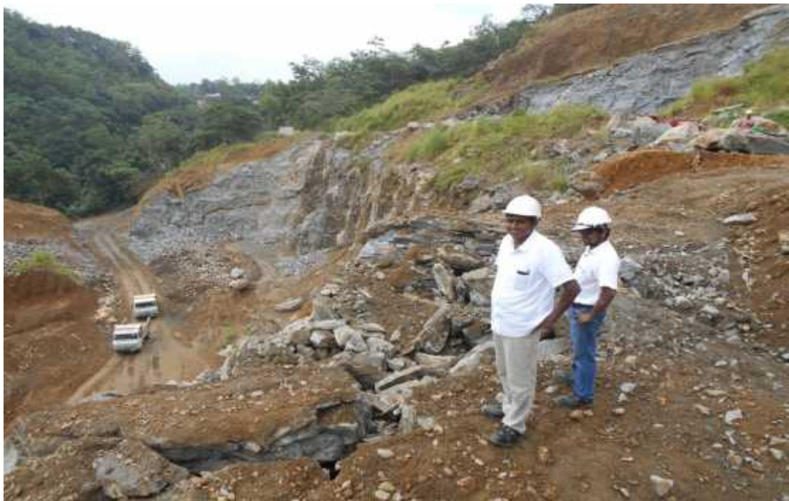
Figure 7.7 After the blast in phase 2
