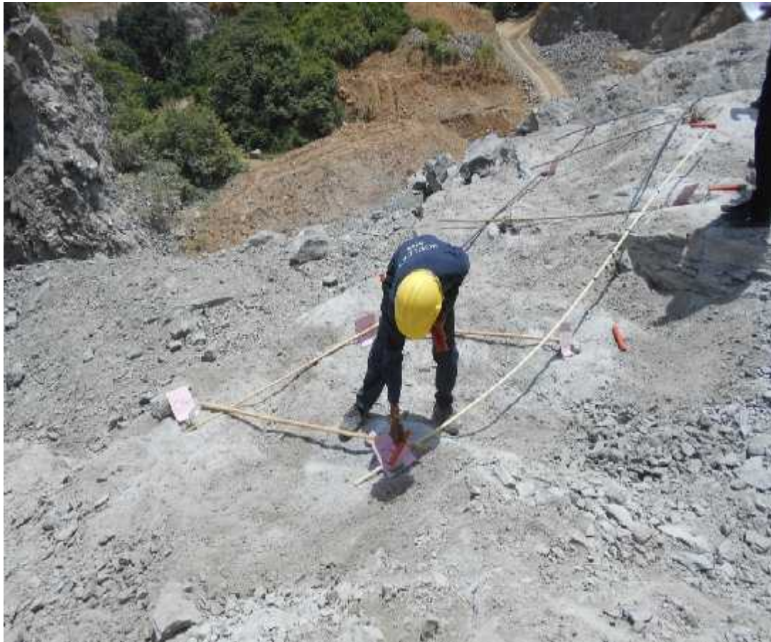
Figure 7.35: Arrangement of bore holes in phase 10
