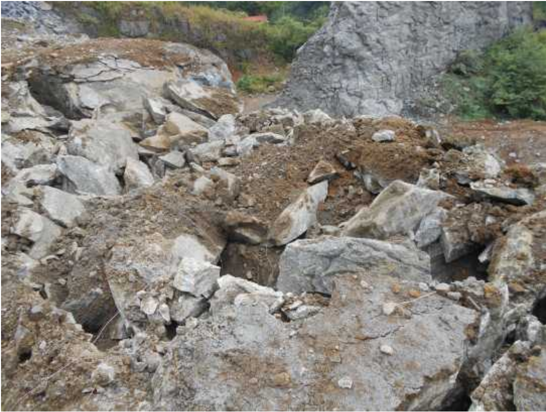
Figure 7.12 After the blast in phase 3
