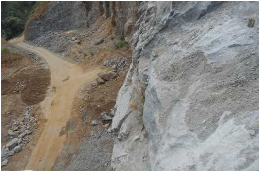
Figure 7.42: cleared area which is expected to receive the products of blasts
