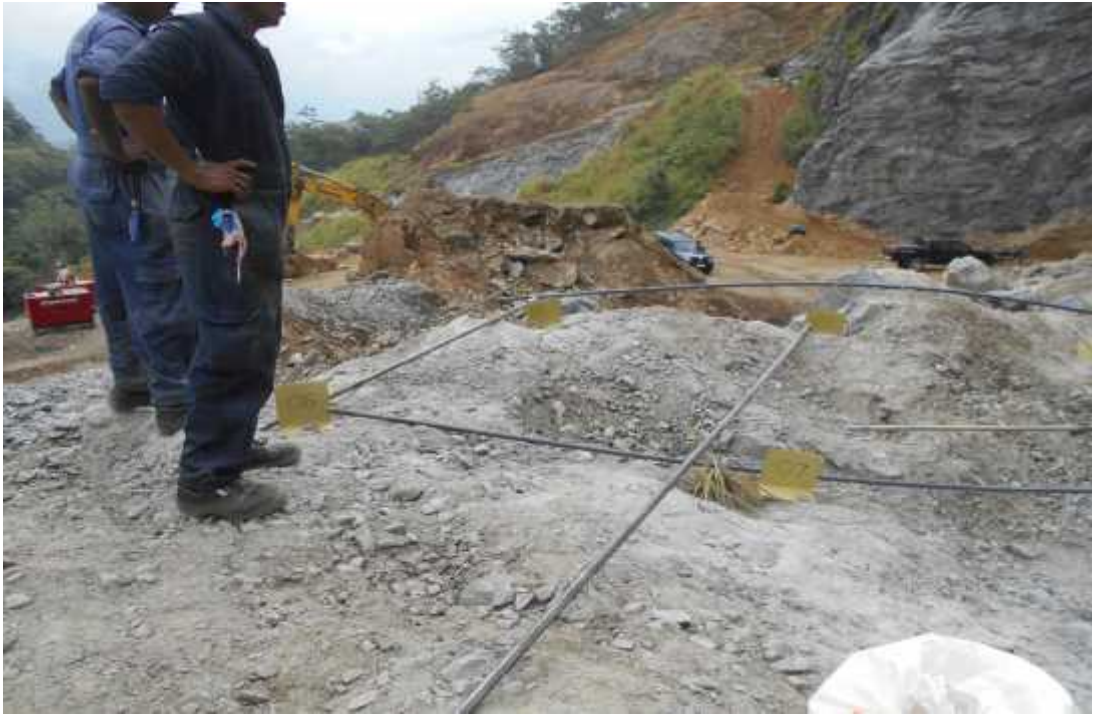
Figure 7.16: Arrangement of bore holes in phase 5
