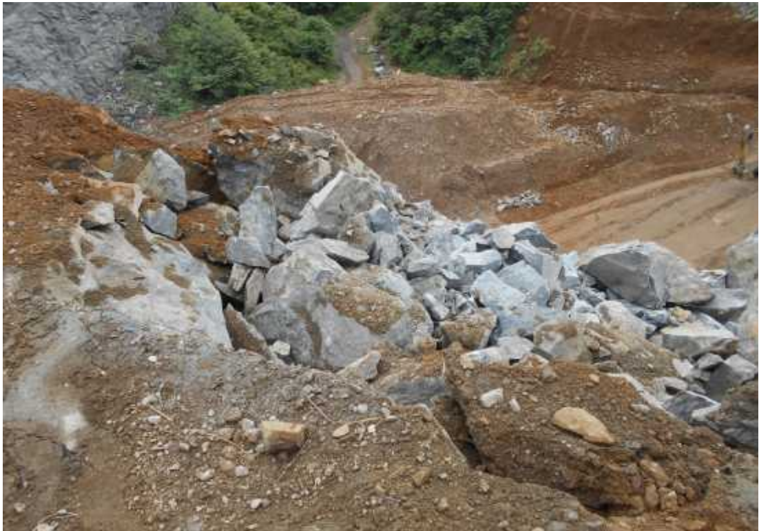
Figure 7.8 After the blast in phase 2
