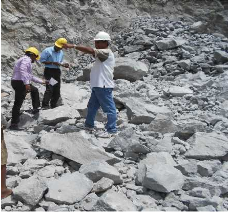
Figure7.32: After the blast in phase 9
