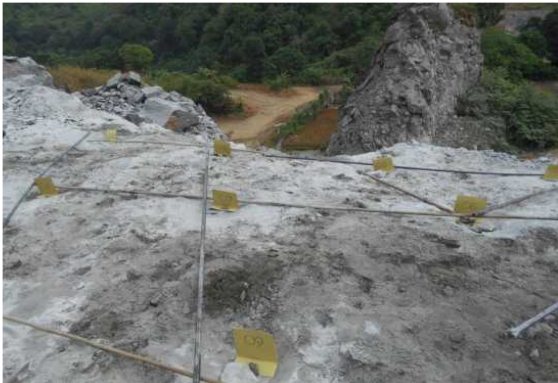
Figure 7.13: Arrangement of bore holes in phase 4
