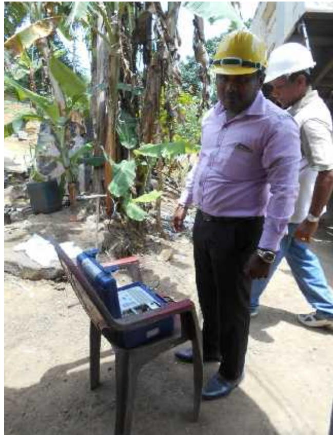
Figure 7.39: Preparing blast mate B for recording
