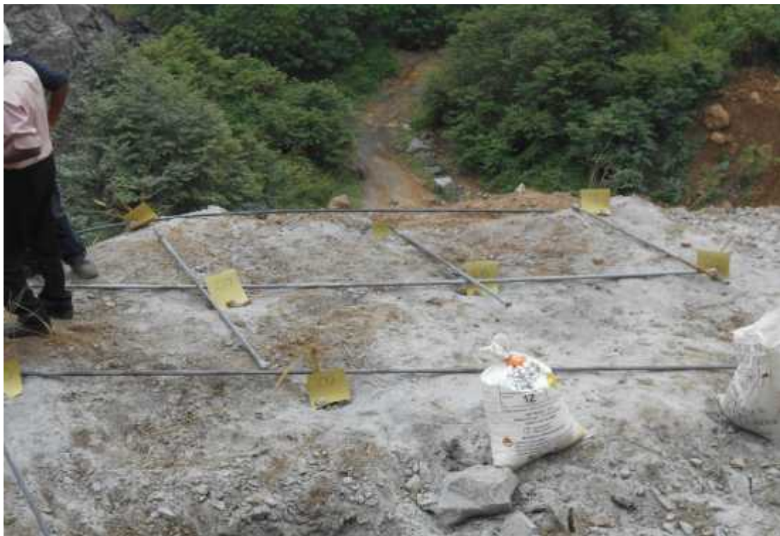
Figure 7.5: Arrangement of bore holes in phase 2
