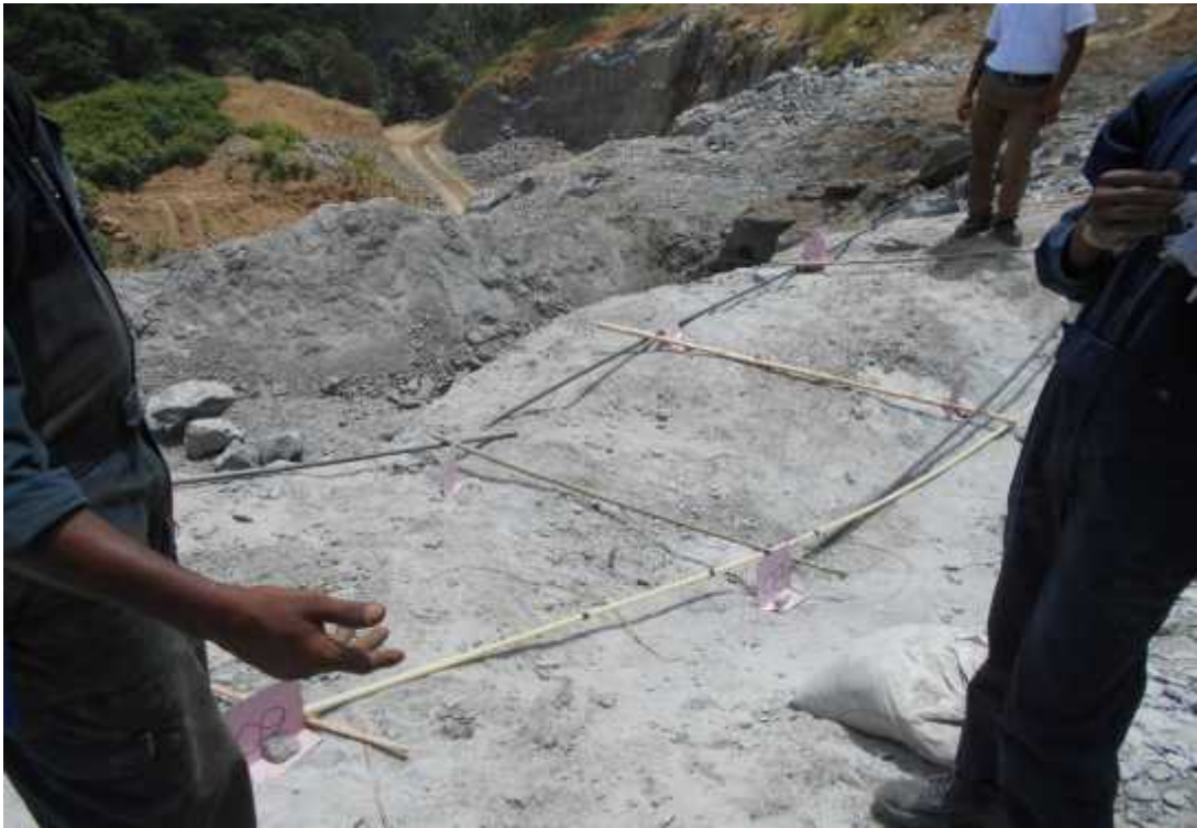
Figure 7.30: Arrangement of bore holes in phase 9
