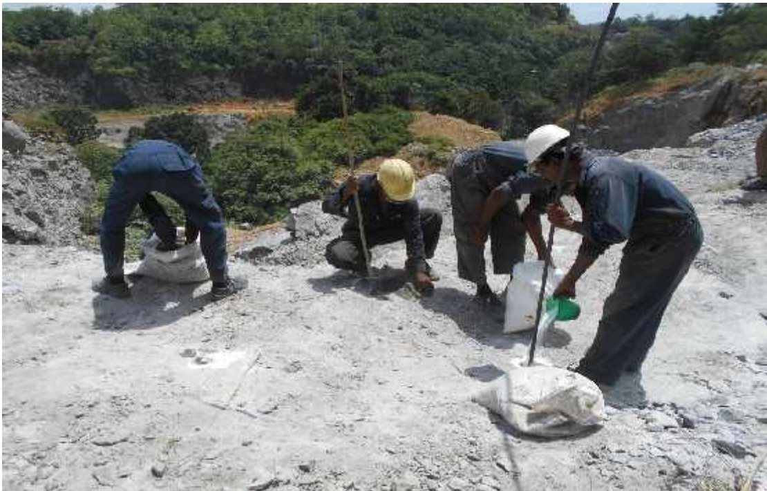
Figure 7.31: Loading of bore holes in phase 9
