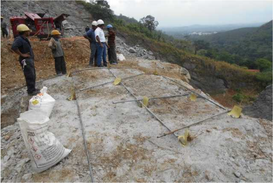
Figure 7.10 Arrangement of bore holes in phase 3
