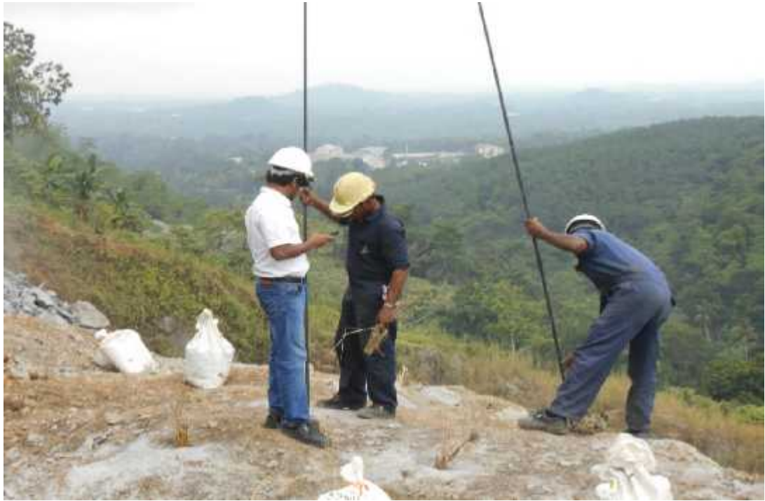
Figure 7.2: Loading of bore holes in phase 1
