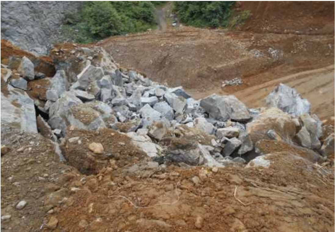
Figure 7.11 After the blast in phase 3
