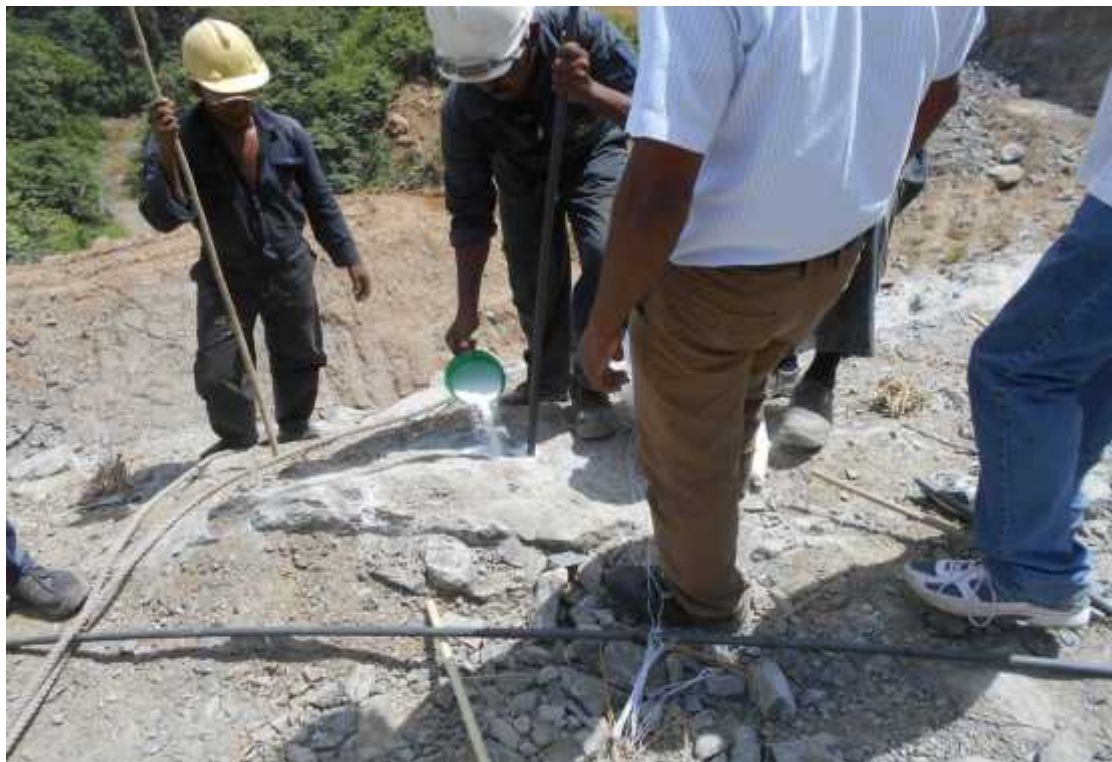
Figure 7.23: Loading of bore holes in phase7
