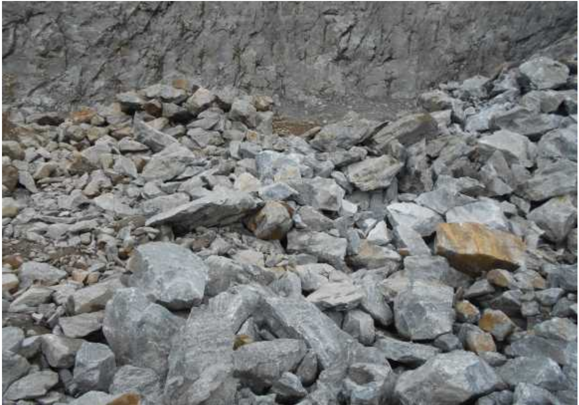
Figure 7.18: After the blast in phase 5
