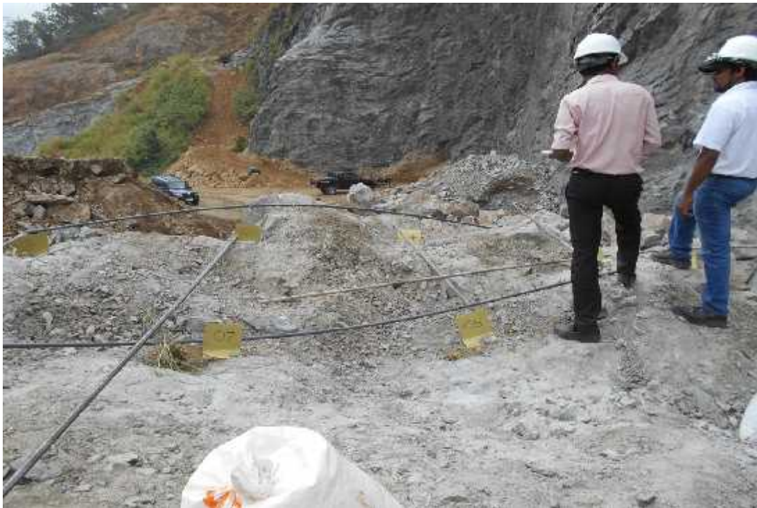
Figure 7.15: Arrangement of bore holes in phase 5
