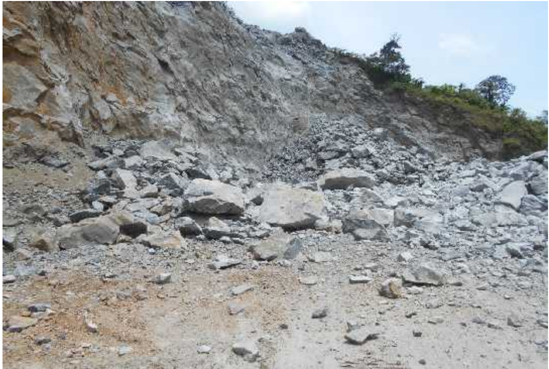
Figure 7.24: After the blast in phase 7
