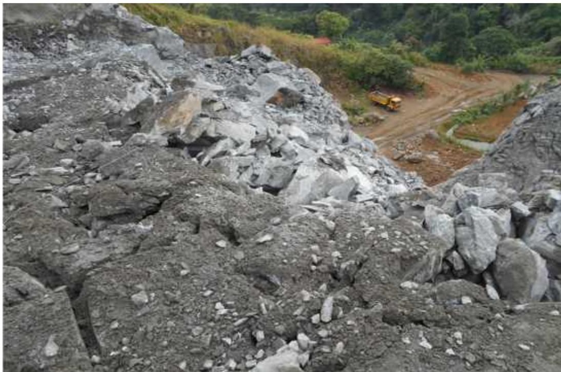
Figure 7.3: After the blast in phase 1
