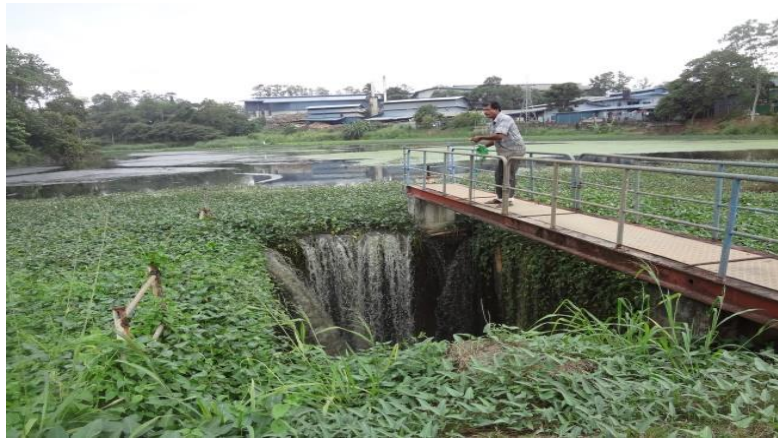
Figure 5. 5 BOI BIP Zone waste water outlet
