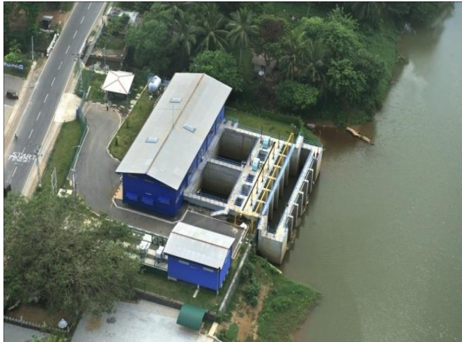
Figure 4.5 Intake Wells, Low lift Pumps and Pumping Main (Source; NWSDB)
