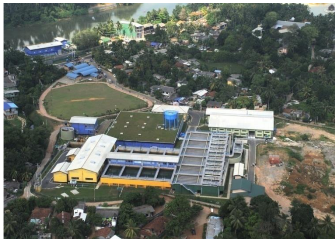
Figure 4.6 Treatment Plant (Source; NWSDB)
