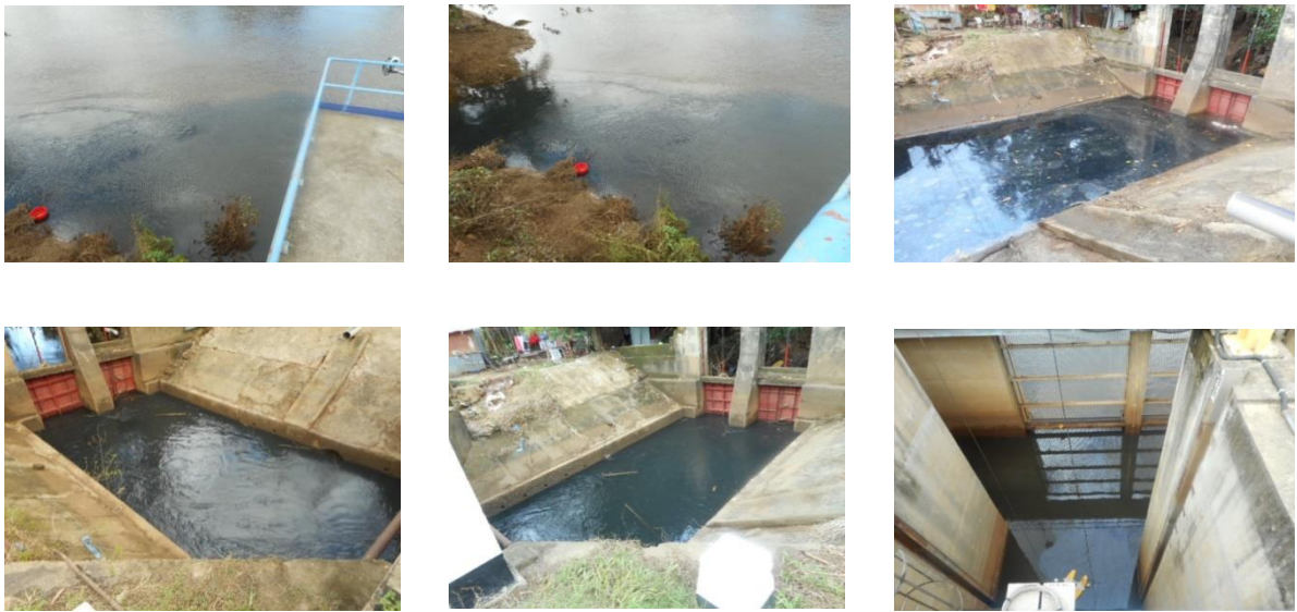
Figure 4.9 Black water visible in Pattiwila canal and Intake on (Source;NWSDB)
