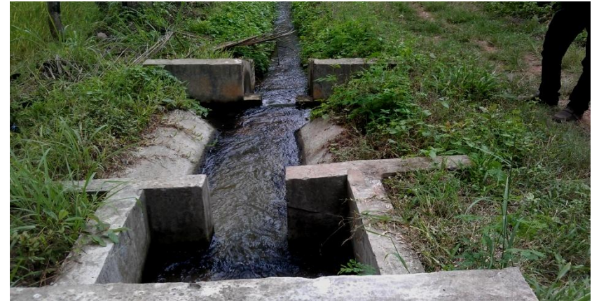
Figure4-7: Field Canal Drop Structure
