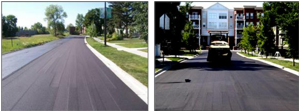
Figure 11: Road Compaction. Left GENCOR HyperTherm. Right GENCOR Foaming
