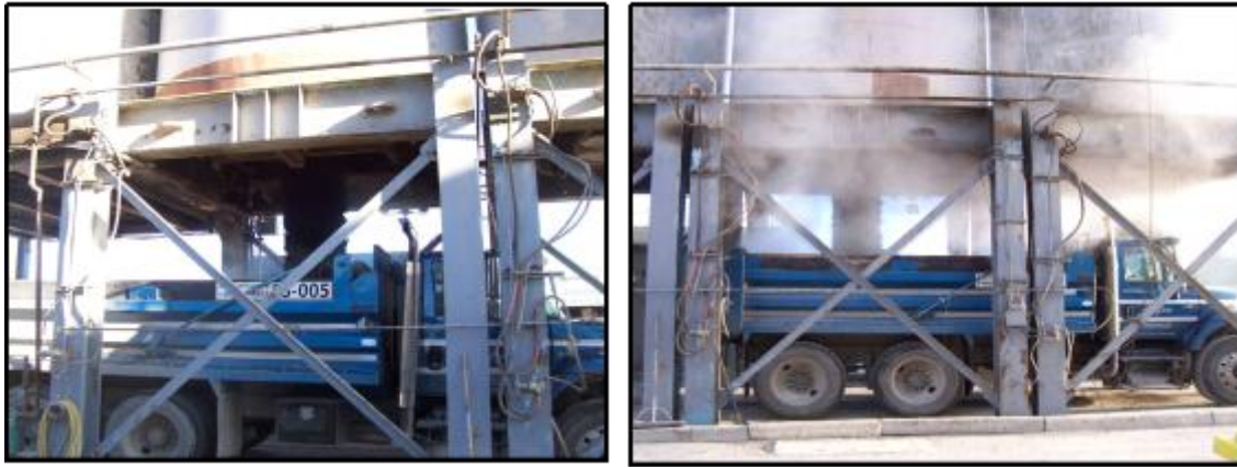
Figure 4: Example of Asphalt Mix Emissions at the Plant. Left GENCOR Foam. Right GENCOR Conventional
