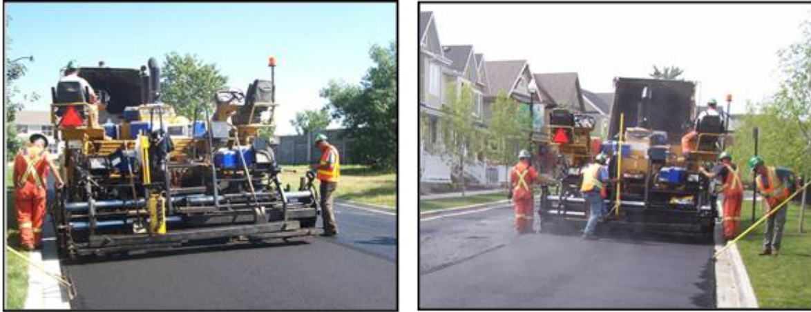
Figure 5: Emission during Road Construction Operations. Left- GENCOR HyperTherm. Right- GENCOR Conventional
