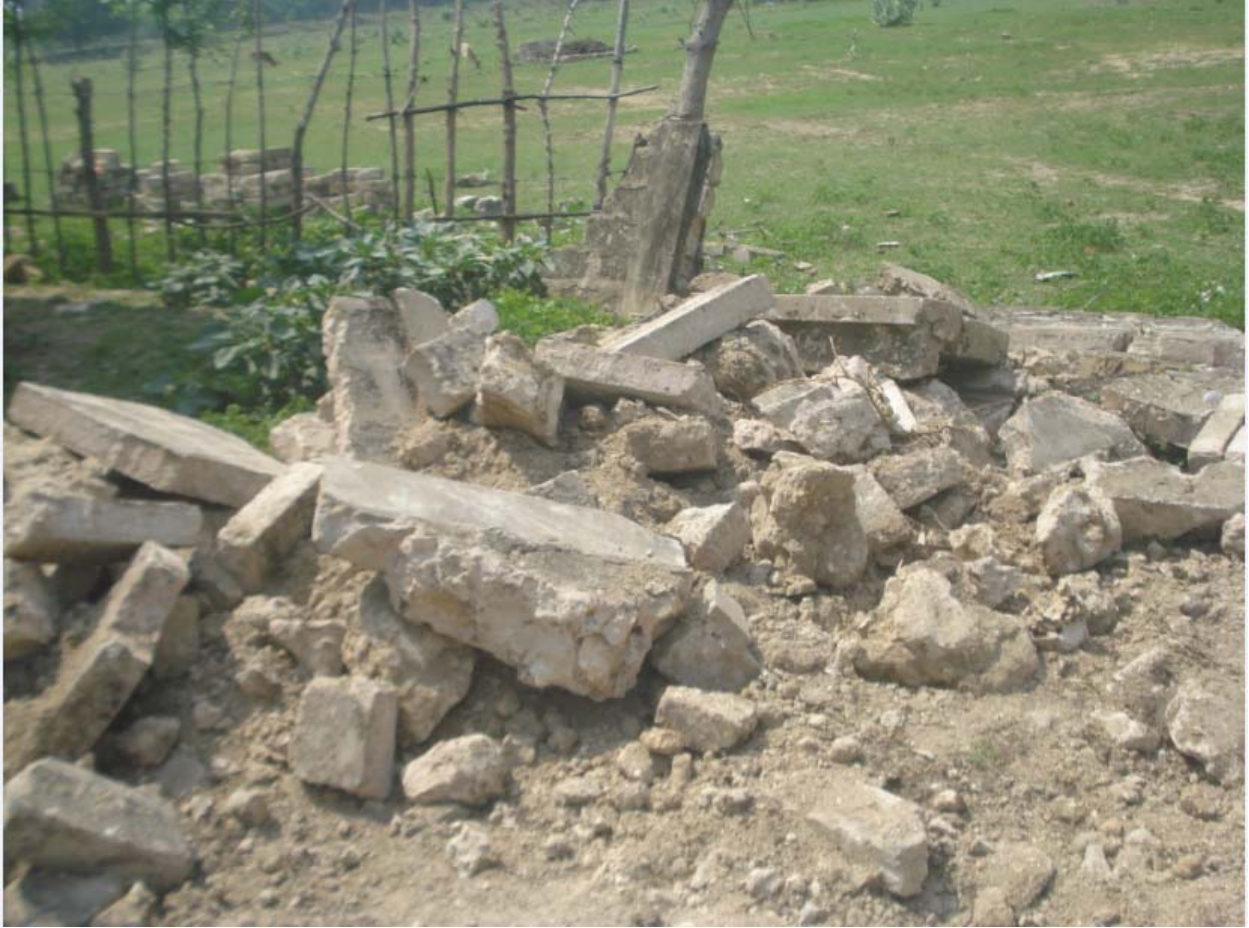
Fig A7.1 (b) Construction Debris
