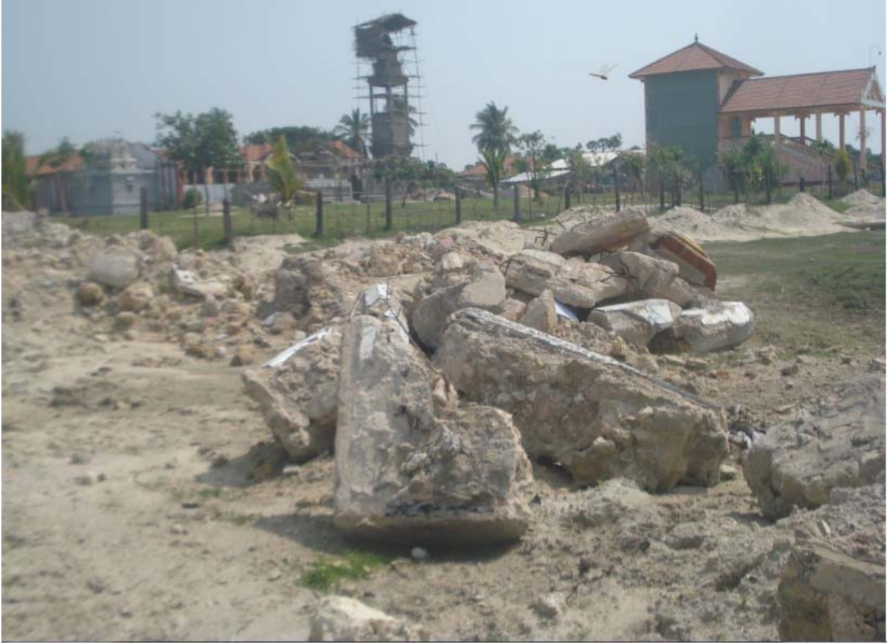
Fig. A7. 2 Concrete Debris
