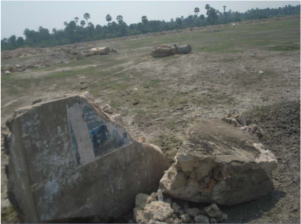
Fig. A7. 1 (a) Construction Debris
