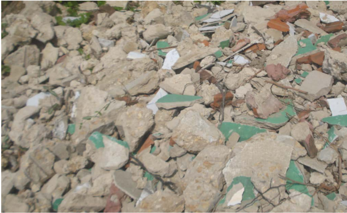
Figure A15.4: Cement Plaster Debris
