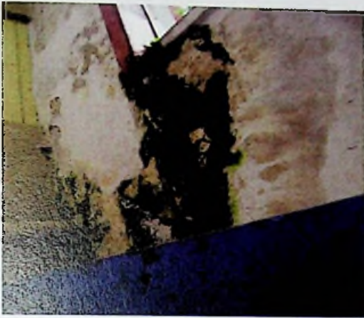
Figure 3. 15: - Fungi and deterioration of wall plasters of OPD Building -LRH
