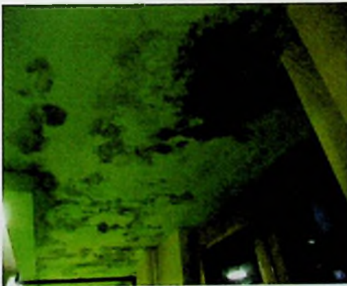
Figure:3.2: formation of fungii,peeling off and blistering of paint at LRH
