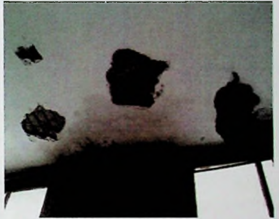
Figure 3.3: Corrosion of reinforcement of slab soffits of OPD building of LRH
