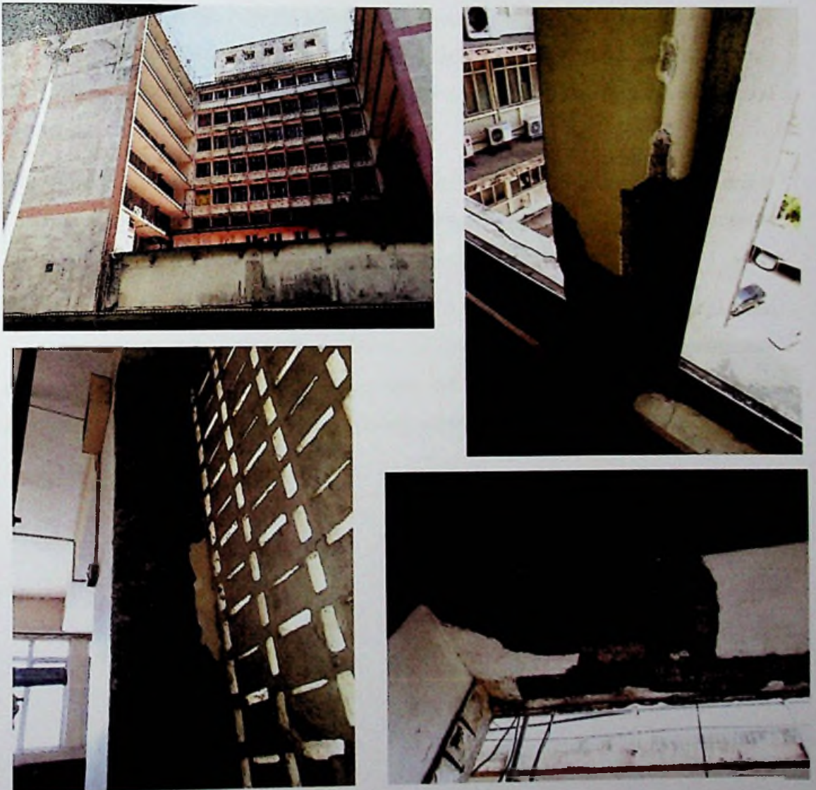
Figure 3.20: Condition of CEB Head Office Building
