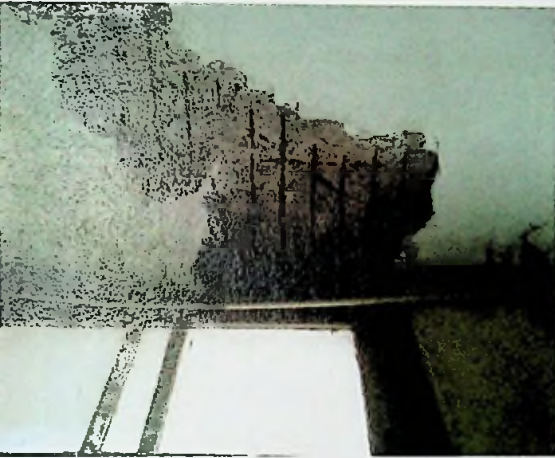
Figure 3.3: Corrosion of reinforcement of slab soffits of OPD building of LRH
