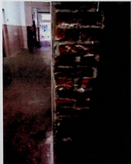
Figure 3.9: Walls of brick masonry in 60 years old OPD building of LRH
