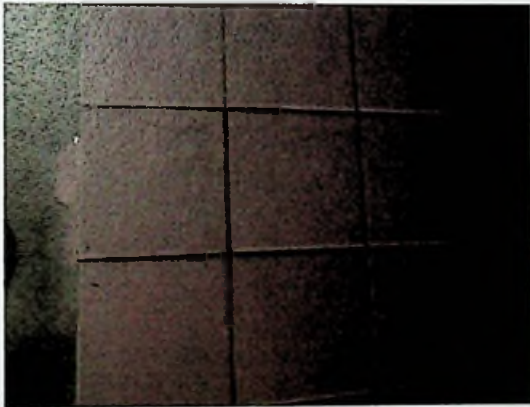
Figure 3.16: Cracks in wall and floor tiles of nine-story building at LRH
