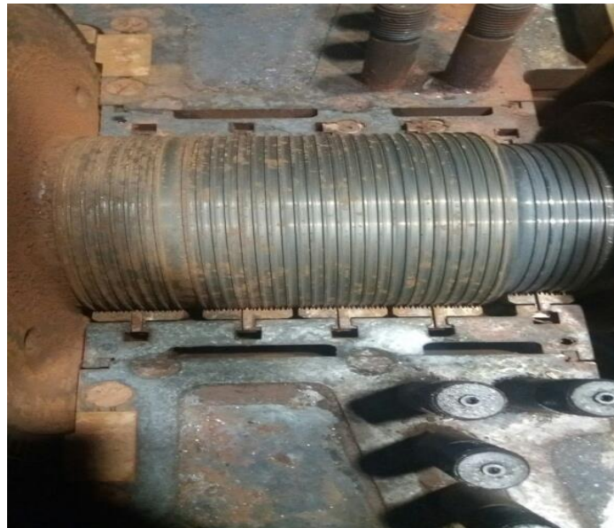
Figure 18: Corrosion at the labyrinth seal
