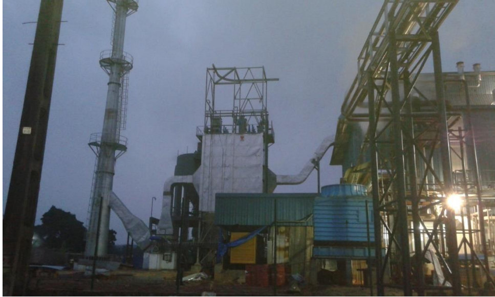
Figure 8: Picture of the Tri-generation Plant
