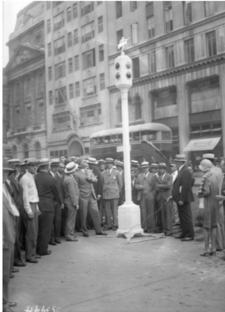
Figure 2-2: Photograph of one of the first traffic signals installed
