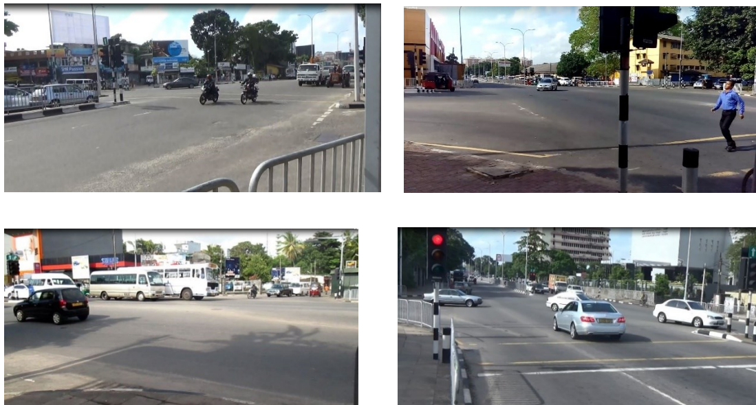
Figure 4-2: Existing Condition of the Baseline Road
