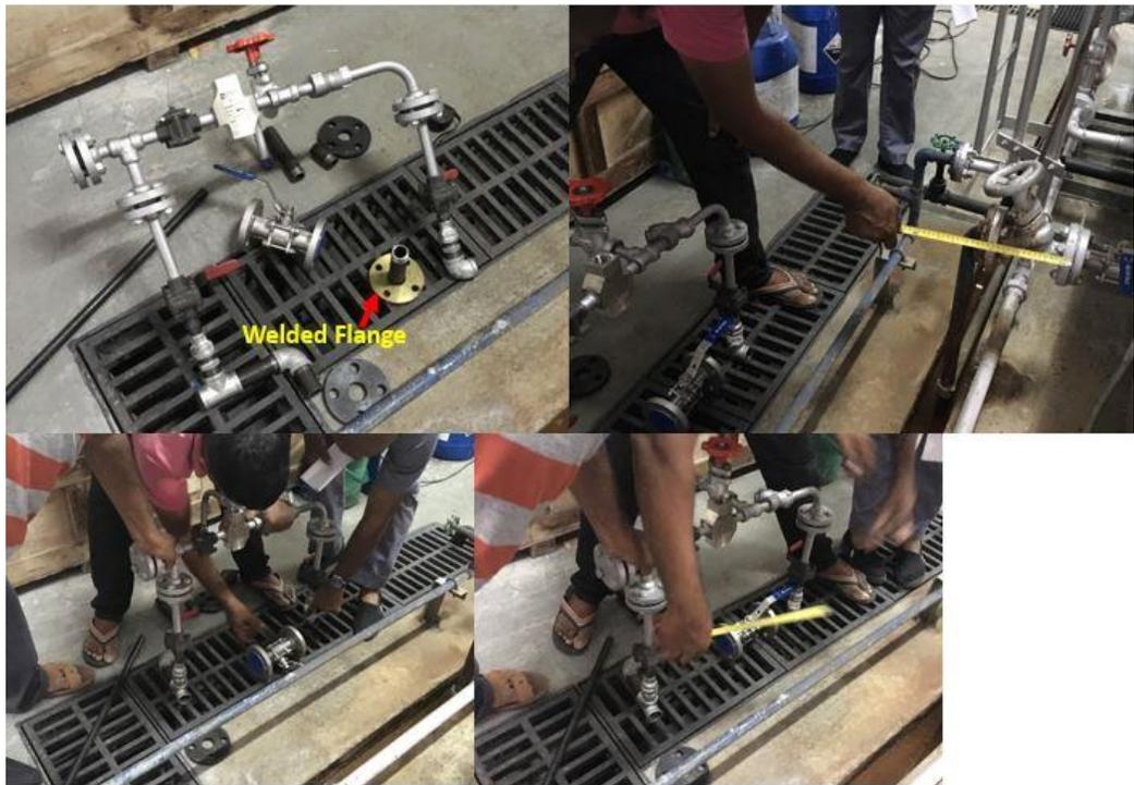
Figure 71: Installation of Design Blowdown Control System
