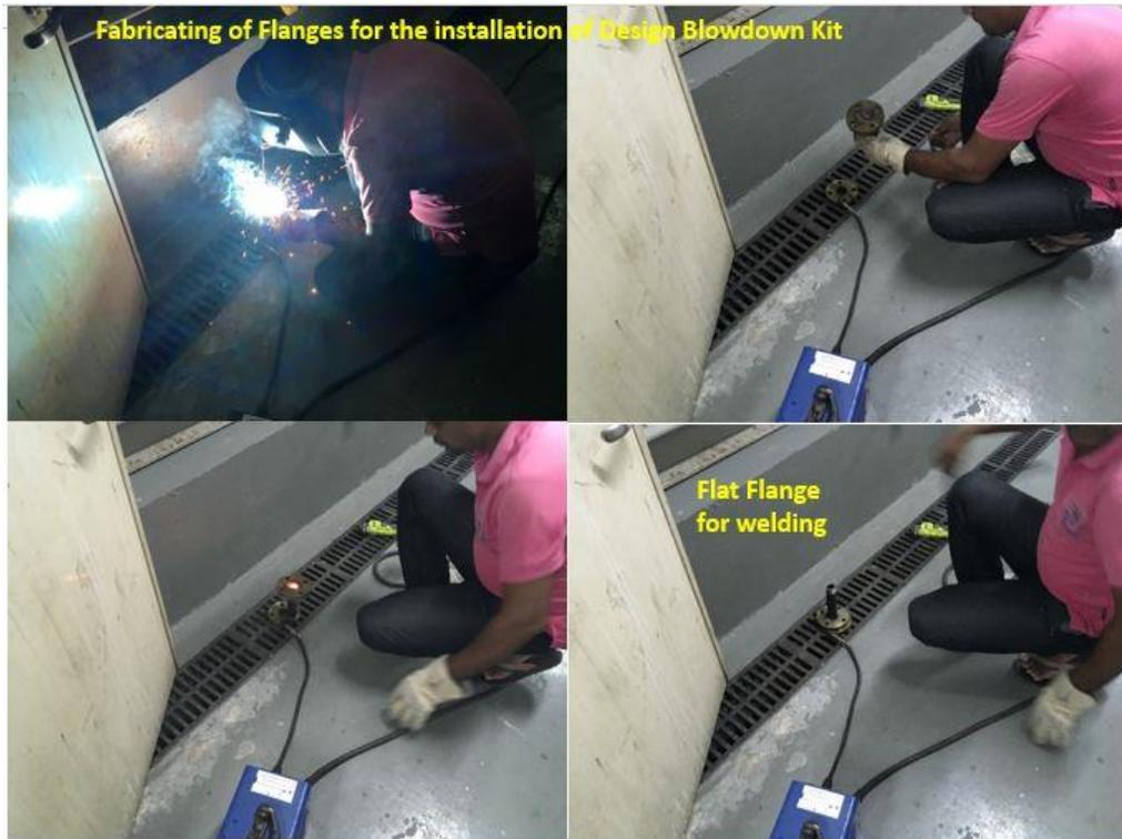
Figure 70: Fabricating of Flanges for Design Blowdown Kit
