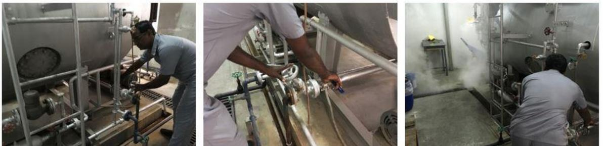
Figure: 18 Manual Blowdown at State Pharmaceuticals Manufacturing Corporation
