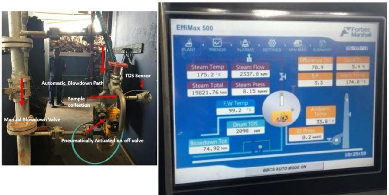
Figure 45: Automatic Blowdown and SCADA System at MAS Biyagama Plant
