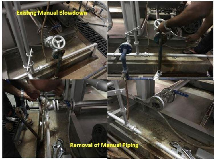
Figure 69: Removal of Existing Manual Blowdown Piping
