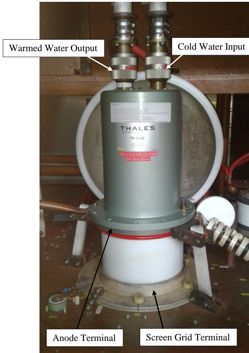
Figure 5: TH558E Electron Emission Tube within the Transmitter
