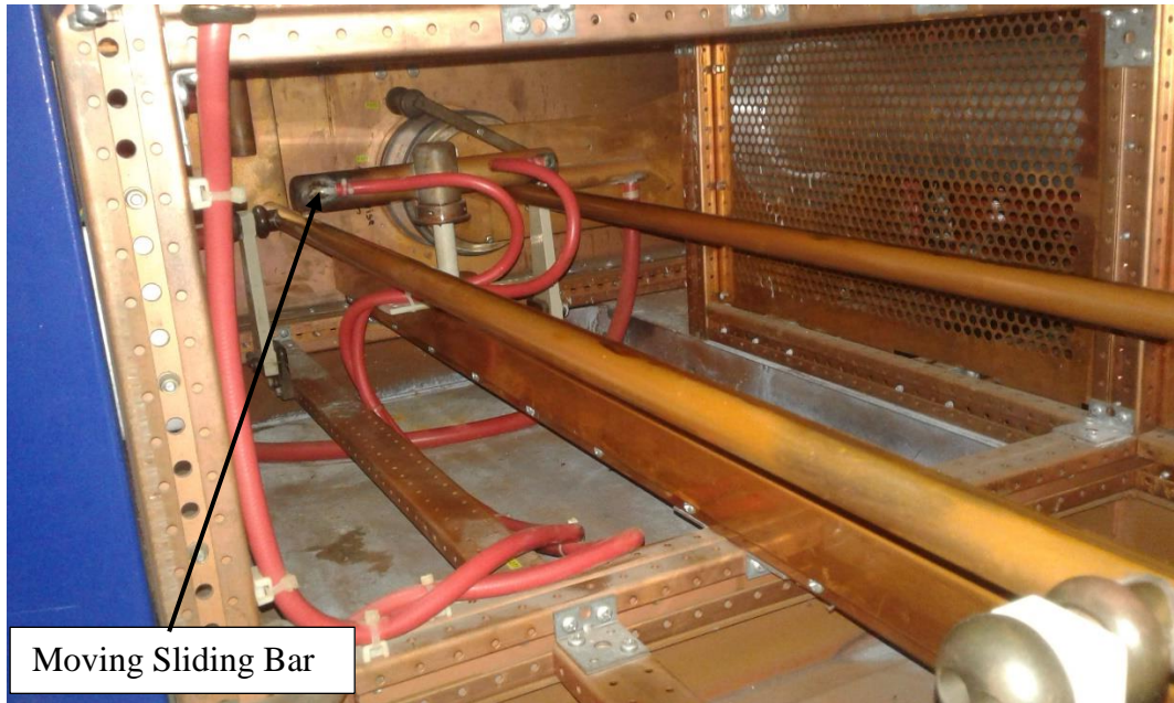
Figure 11: Moving Sliding Bar for Varying the Inductance
