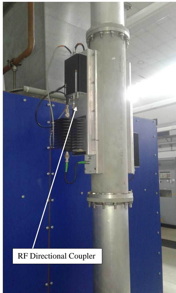
Figure 4: RF Directional Coupler for Measuring Output RF Power
