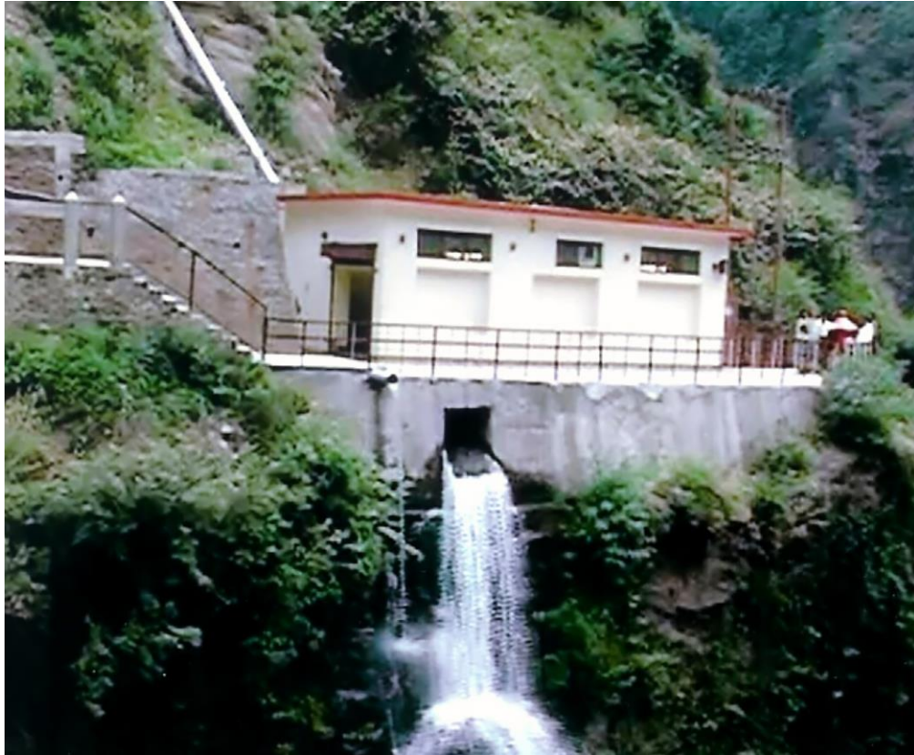
Fig 2. A small Hydro Power station
