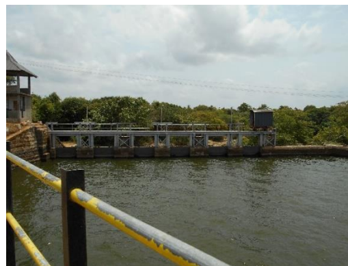
Figure A.4: Gated Spillway (original in colour)
