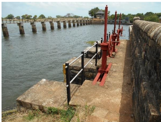
Figure A.9: RB Low Level Sluice (original in colour)
