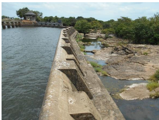
Figure A.3: Un-gated spillway (original in colour)
