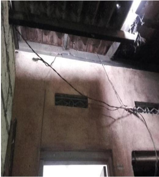
**Figure 4-11 Insecure wiring in
