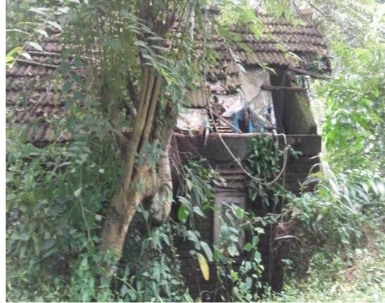
**Figure 4-12 Collapse of roof due to improper maintenance Arahena**
