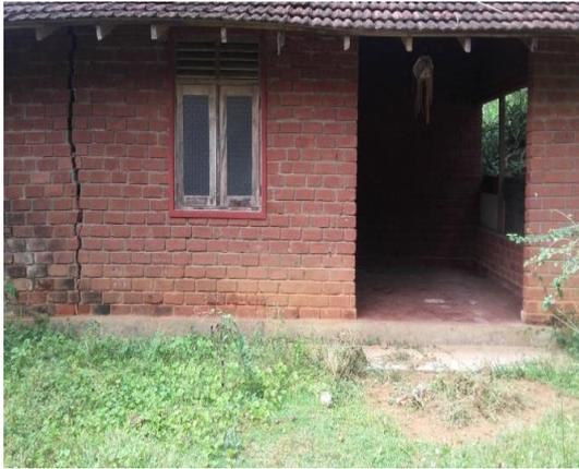
**Figure 4-13 Crack on wall. This house is abandoned due to Unlivable condition in Arahena Matara**
