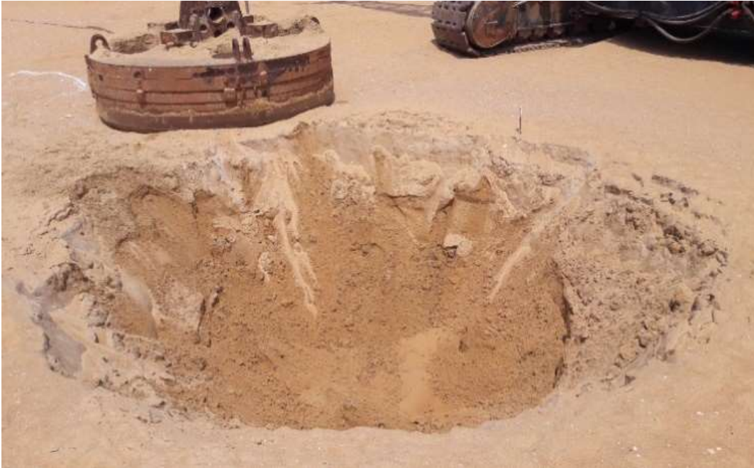
Figure 4-17: typical crater seen during dynamic compaction
