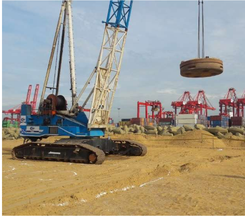
Figure 4-11: Application of dynamic compaction
