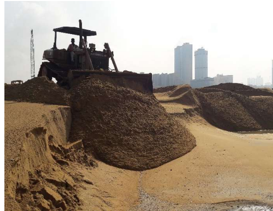
Figure 2-4: Sand dumping and moving by earth movers
