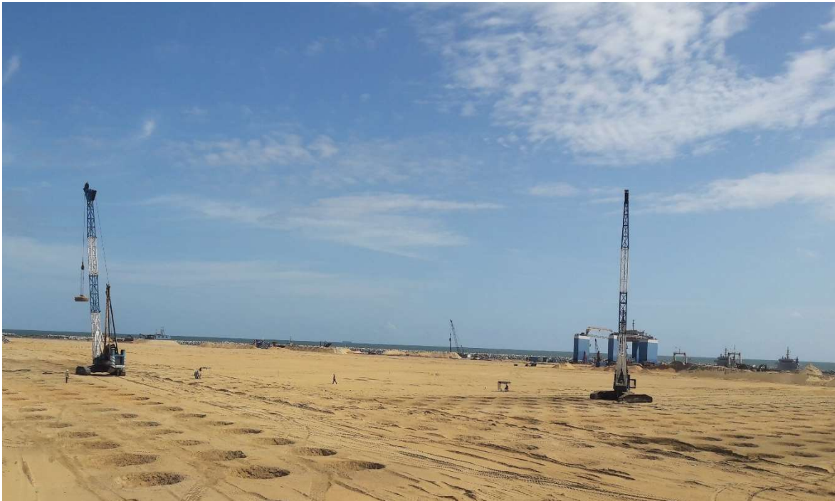
Figure 2-24: Dynamic compaction done in the project site
