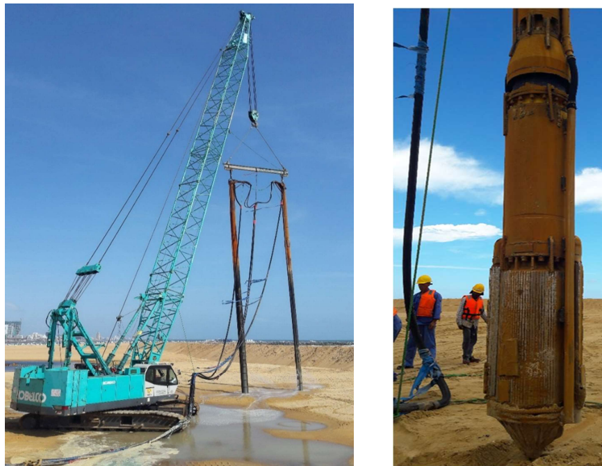
Figure 2-28: Vibro Compaction done in Project Area
