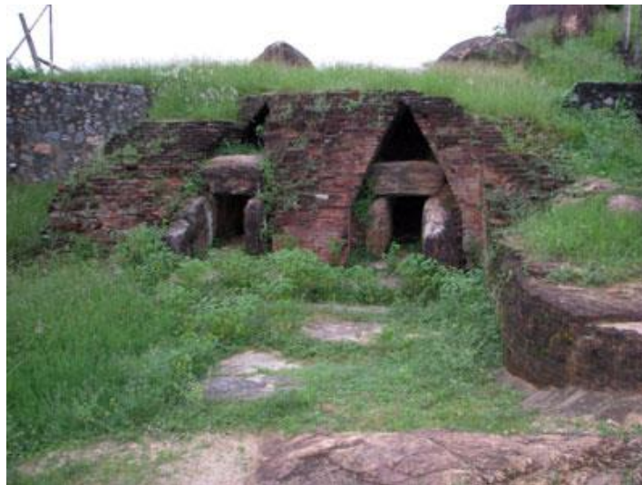
Fig.1.5 Ancient Maduru Oya Sluice of 1 st century BC
