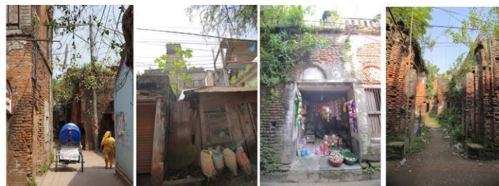
Figure 8, Images from road representing poor conditions. (Source: Author)
