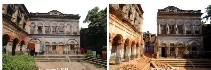
Figure 5, Demolition of house 3 in 2017 (Source: Author)
