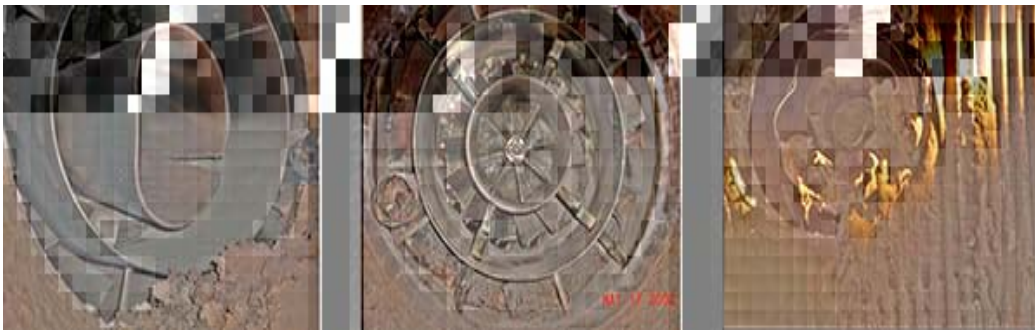
Figure 2. 1: Slagging and fouling problems in boilers
