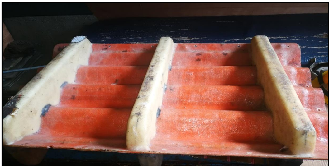
Figure 4.3: Plug Preparation Complete
