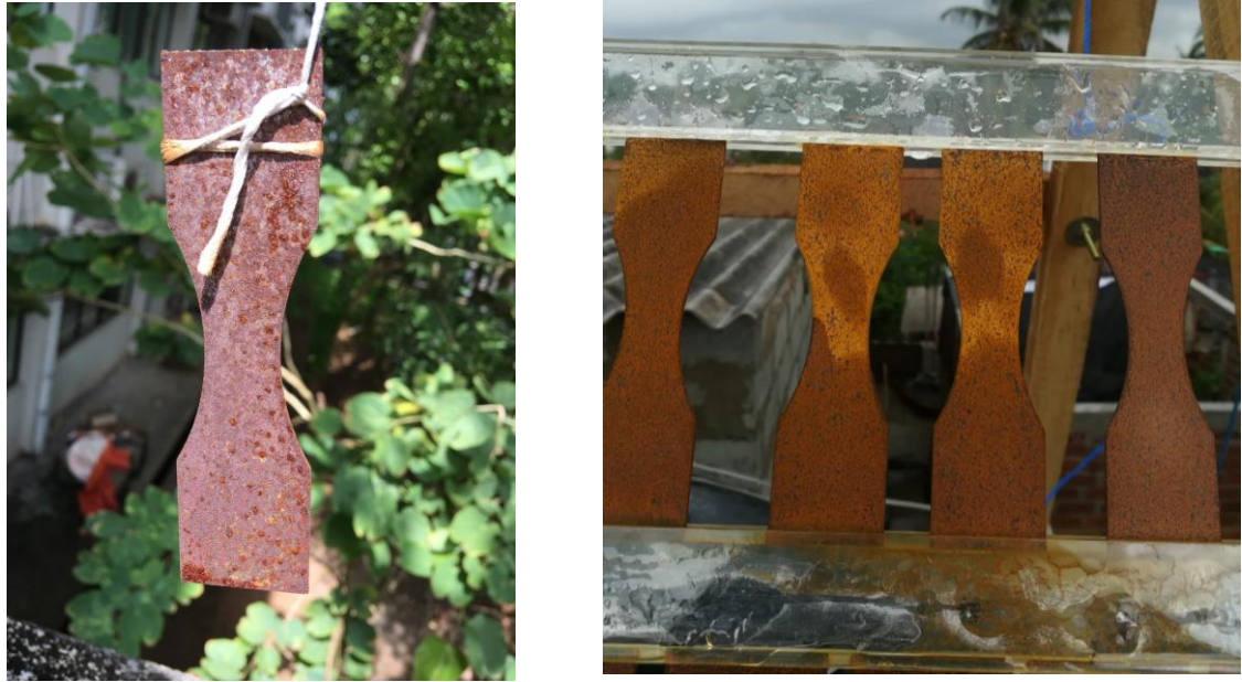
Figure 3. 22 : Even corrosion in environmental conditions
