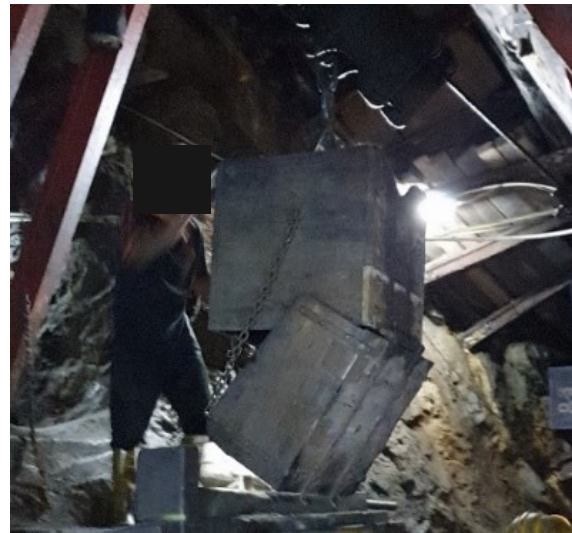
Figure 4: Unloading from 'Winch Box' at Kahatagaha mine.
