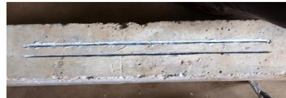
Fig. 2 Grooves prepared parallel to main reinforcement (at the bottom face)
