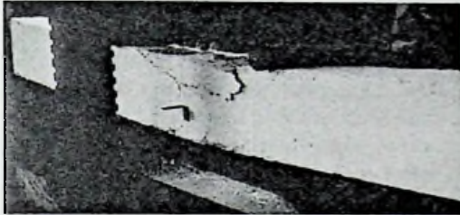
Figure 3: Failure of beam with shear links
