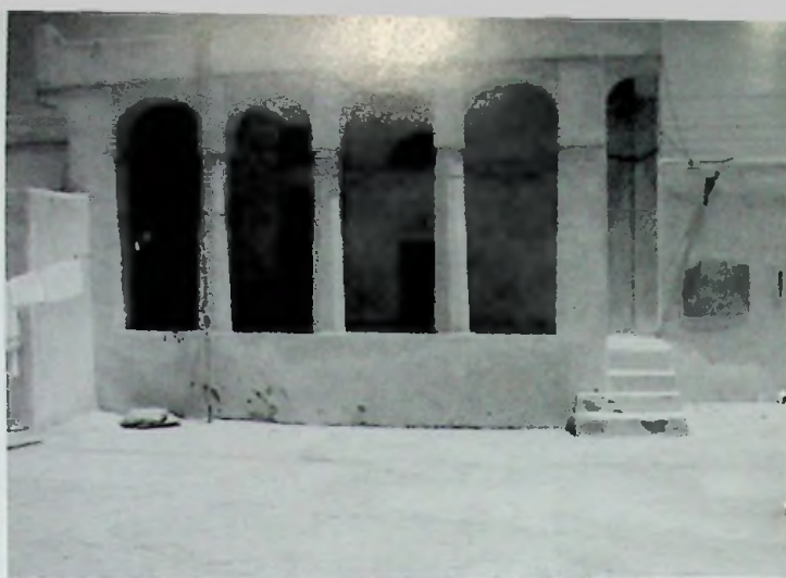
Figure 7: A mozif in a vernacular house
