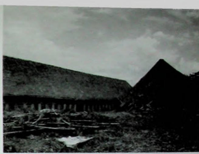
Figure 12: Jember's Los totally damaged by wind storm. Source: Author's documentation, 2010.
