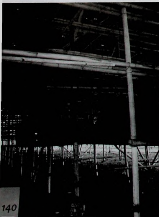
Figure 15: Jember's Los with iron columns erected on concrete foundations. Source: Author's documentation, 2010.
