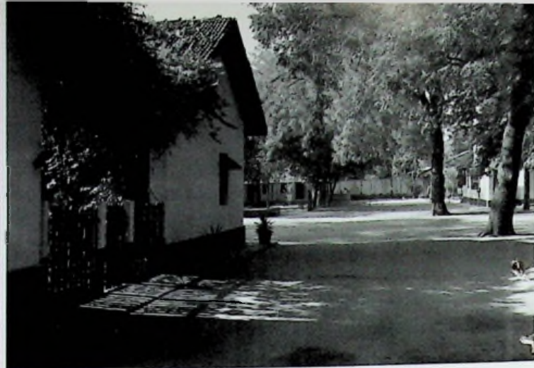
Img 2: Ashram Side Entry Into Hruday Kunj
