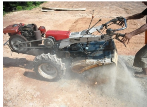
Figure 3.3 : Rotary mixing in field
