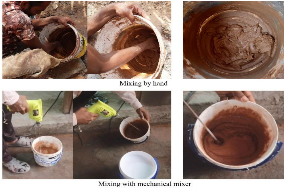
Figure 7.27: Mixing the sludge putty mixture
