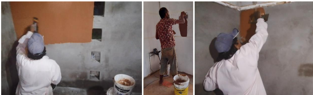
Figure 7.28: Sludge putty application on wall plaster
