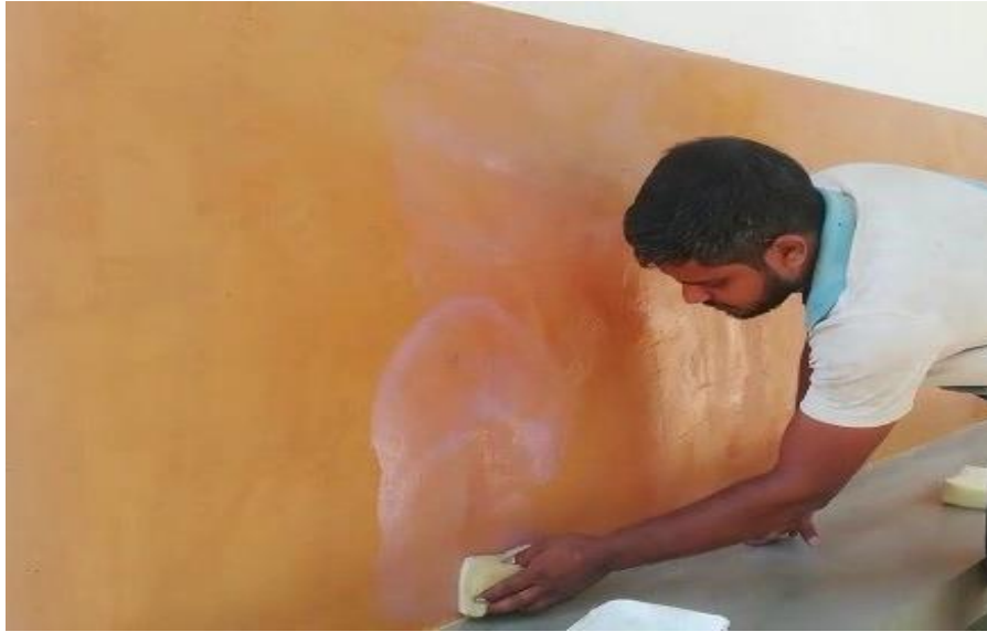
Figure 7.31: Applying sealer on sludge putty surface as a top coat
