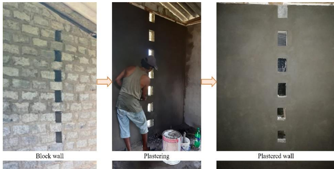
Figure 7.26: Wall preparation for putty application
