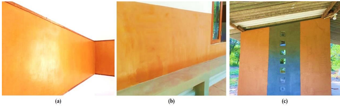
Figure 7.32: Selected sludge putty applied walls to analyze performances; (a) Interior wall (b) exterior wall (c) Exterior wall with shade
