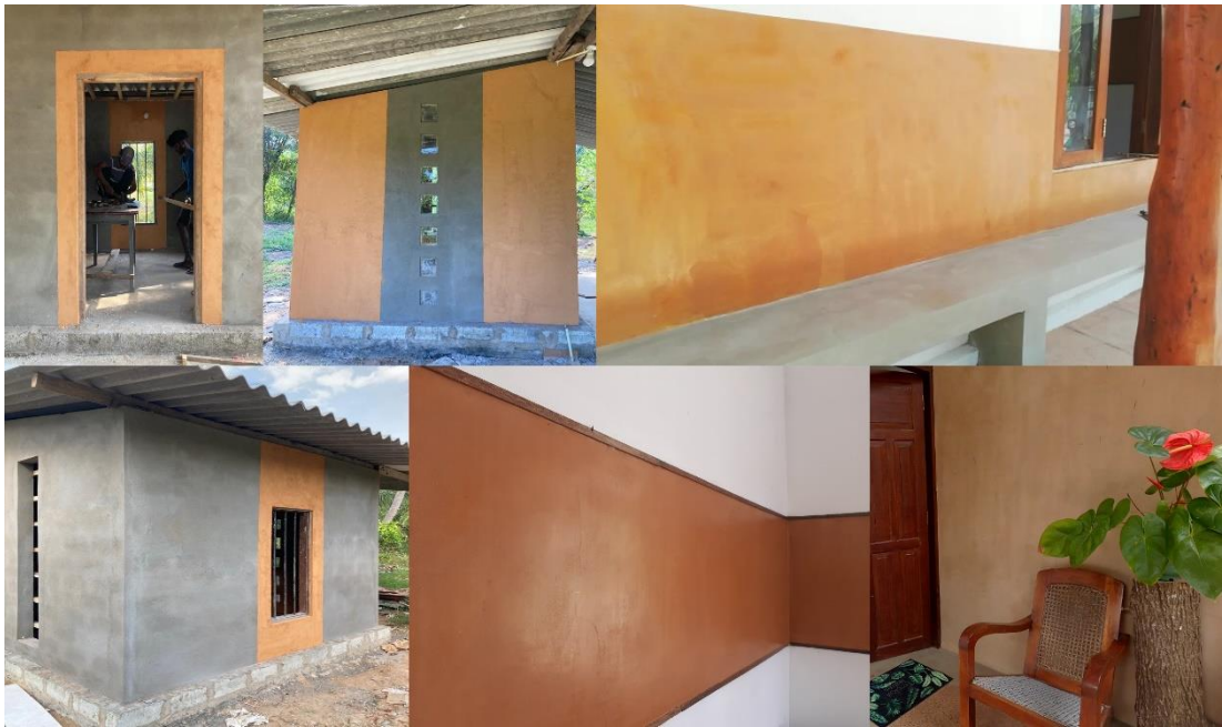
Figure 7.23: Real-scale applications of the sludge putty
