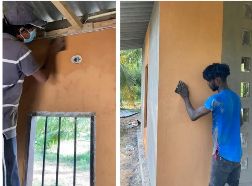
Figure 7.30: Sanding the putty surface with sandpapers
