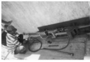
Post stressing the dome using stainless steel cables
