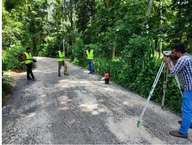
Figure 7.5 level reading at 1 m interval before asphalt laying
