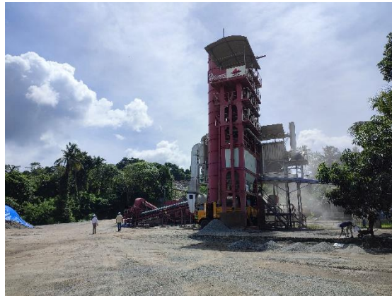
Figure 7.1 Kotadeniyawa asphalt plant
