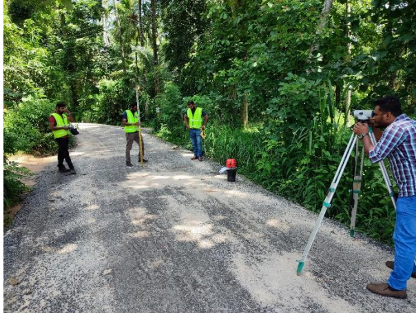
Figure 2.1 Level survey prior laying asphalt layer
