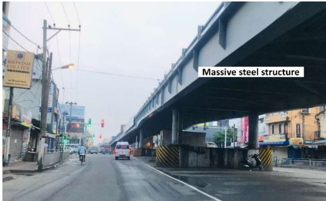
Figure 21: Dehiwala Flyover Source: Compiled by Author
