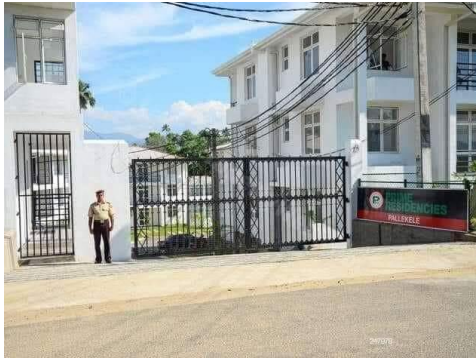
Figure 8: Entrance of Prime Residences Source: Broacher of Prime Residences, 2017
