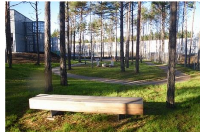
Figure 17 -Halden prison: Boundary wall as seen from the interior [Online image] (Source: http://www.gossiprocks.com )
