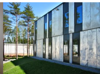
Figure 20 -Halden prison: Exterior view of accommodation blocks [Online image] (Source: www.moma.org )
