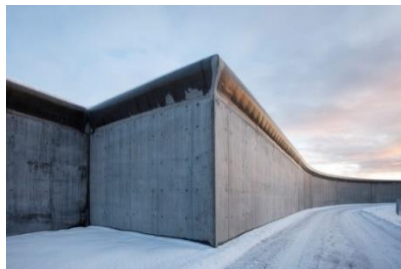
Figure 16 -Halden prison: Boundary wall [Online image] (Source: www.moma.org )
