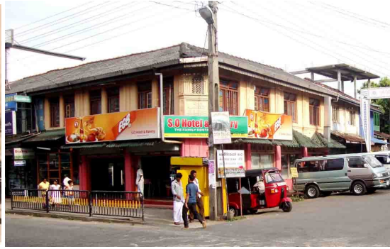
Figure 33: S.O Hotel building (1944), Mawanella - 2013 Source: Author
