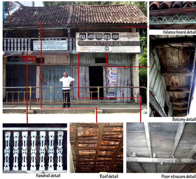
Figure 14: Scale, proportion, appearance and direction of built components generated to accommodate slow, light traffic – First stage development Source: Author
