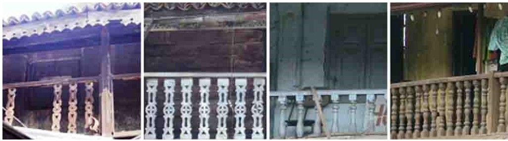
Figure 36: Decorative building façade reveal personalization Source: Author
