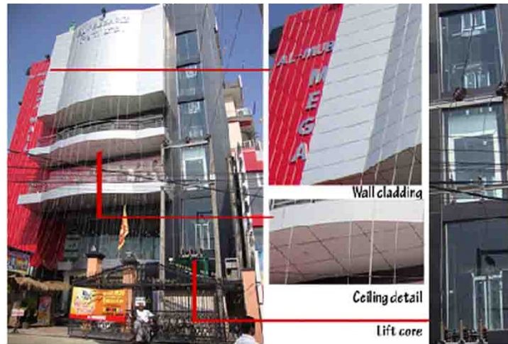
Figure 16: Variety of building components – Third stage of stage development (Constructed at the end of stage) Source: Author
