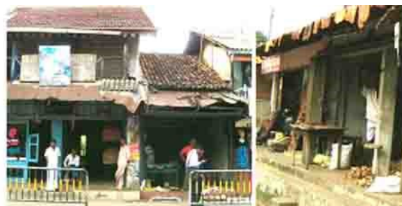
Figure 24: Multi-functional front verandah in old shop houses Source: Author
