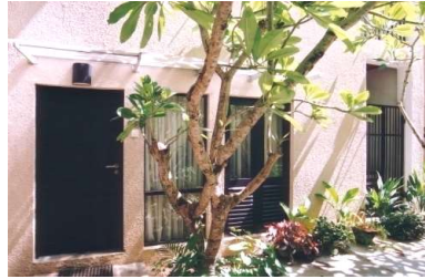
Fig 23 - Ground floor units' connection with pathway. Source- Sierra Property Developers (Pvt). Ltd
