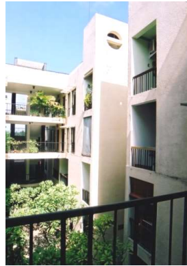
Fig 15 - Balconies are mainly focused towards the middle courtyard – Case 1 Source- Sierra Property Developers (Pvt). Ltd
