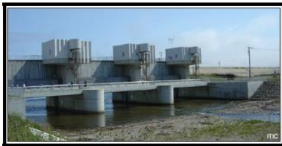
Figure 30: Water Gates, Okushiri Island, Japan. [53]
