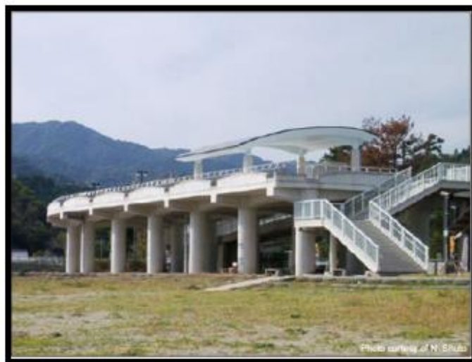
Figure 28: an elevated shelter at Shirahama, Tokushima Prefecture, Japan
