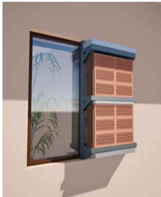
Figure 04: Hybrid system featuring terracotta for dehumidification developed by Team Solstice (Team Solstice, 2024)
