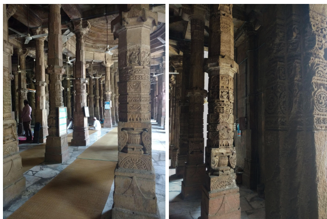
Figure 3. Columns placed on each other to achieve the desired height of the mosque. The figures are sourced from the author.
