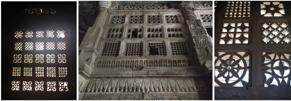
Figure 5. The jalis were used to control light and create the zanana in the mosque. The figures are sourced from the author.
