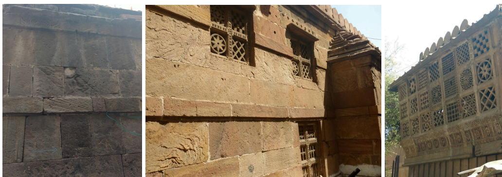
Figure 1. The structure is built with pillaged material. The figures are sourced from the author.
